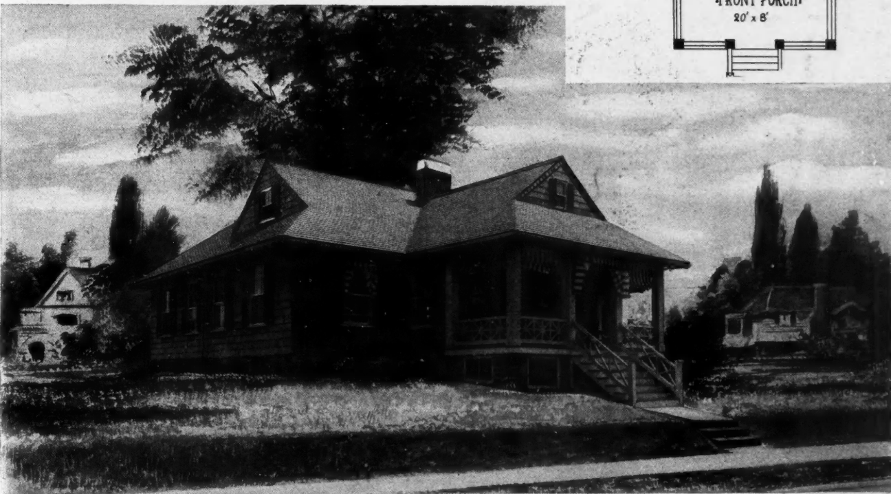
Cozy little bungalow of five rooms. Size, 40 feet by 34 feet 6 inches. We can furnish complete set of blueprinted working plans and typewritten specifications for only $6.00 per set. Blueprints consist of basement plan; roof plan; main floor plan; front, rear, two side elevations; wall sections; and all necessary interior details. Specifications consist of twenty-two pages of typewritten matter. When ordering, ask for Design No. 6743.
