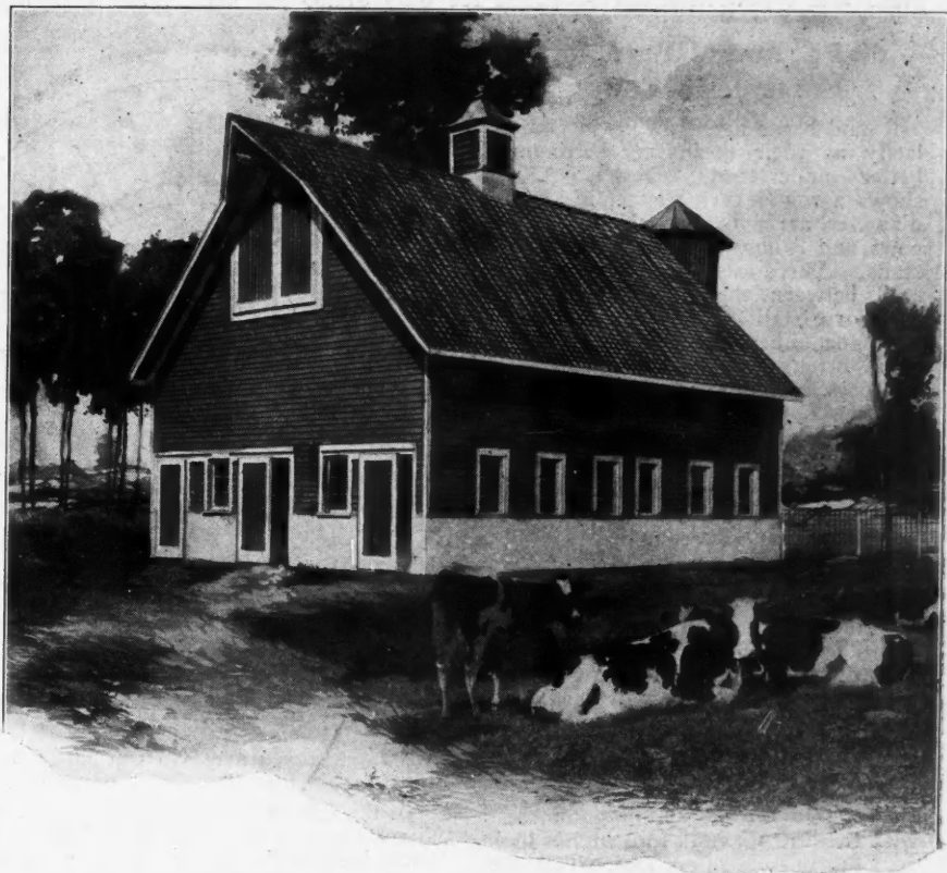
Gable roof horse and cow barn with high concrete foundations, size 48 by 34 feet. Arranged for thirteen cows and eight horses. We can furnish complete set of blue-printed working plans and typewritten specifications for only $7.00 per set. When ordering ask for Design No. A335.
