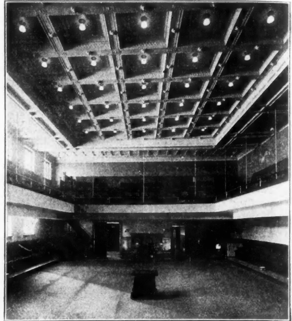
I. O. O. F. Lodge Room, Des Moines, Iowa, with Newly Installed "Classik" Steel Ceiling.
