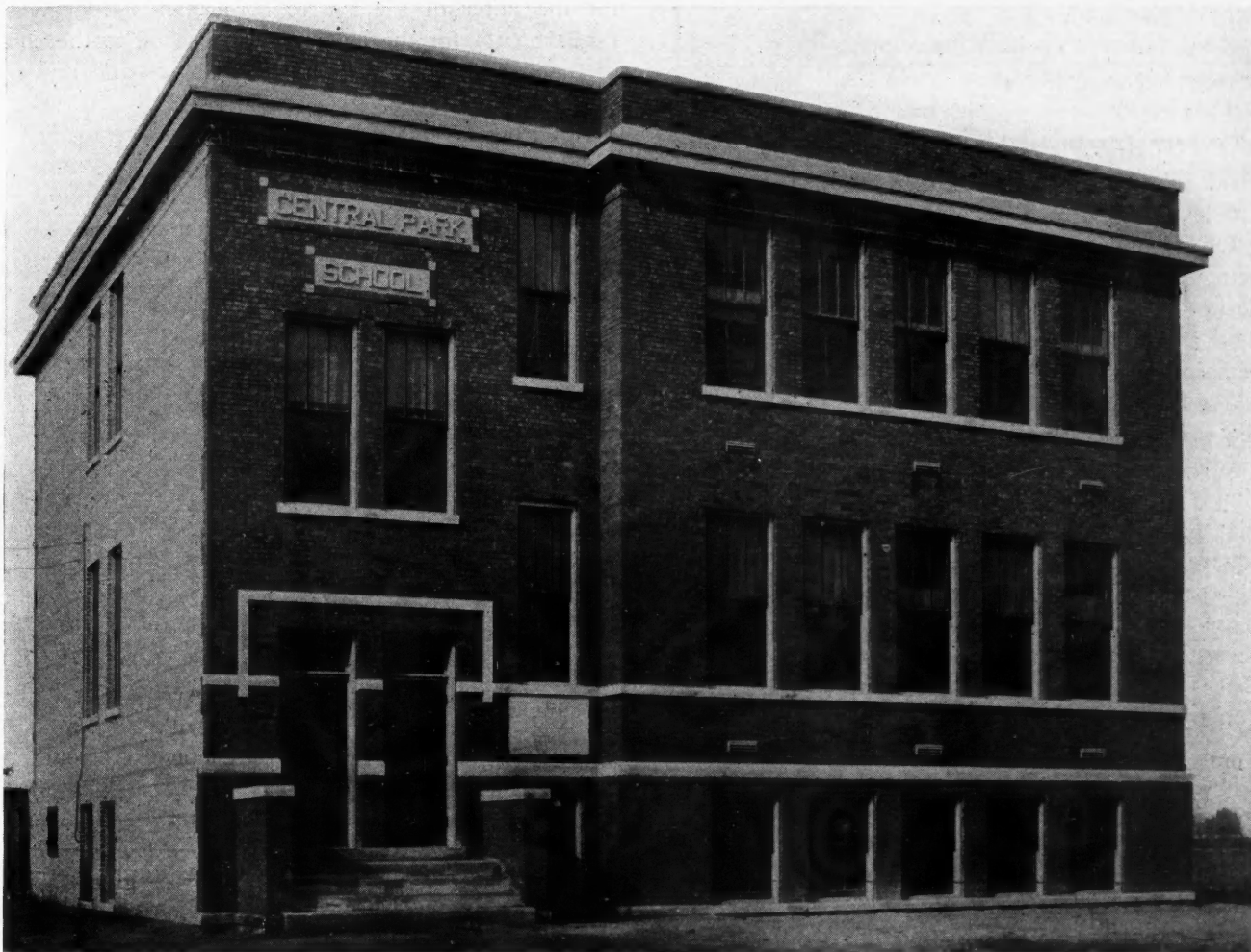
First Half of Central Park School, Mt. Greenwood, Ill. Designed by the Well-known Schoolhouse Architect, G. W. Ashby.
