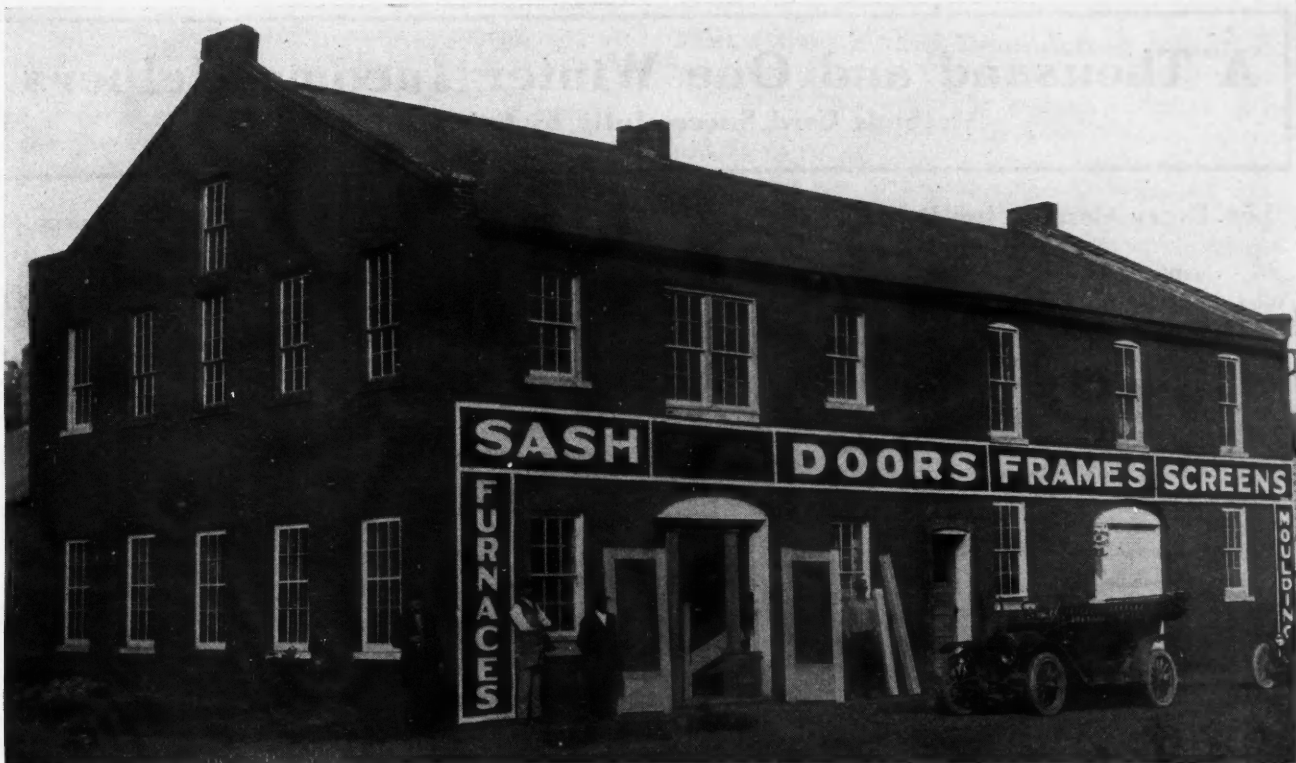
The Marsh Shop is Two Stories, Size 70 by 85 ft. Used as Headquarters for His Various Special Contracting Crews, that Handle Anything and Everything in the Building Line.
