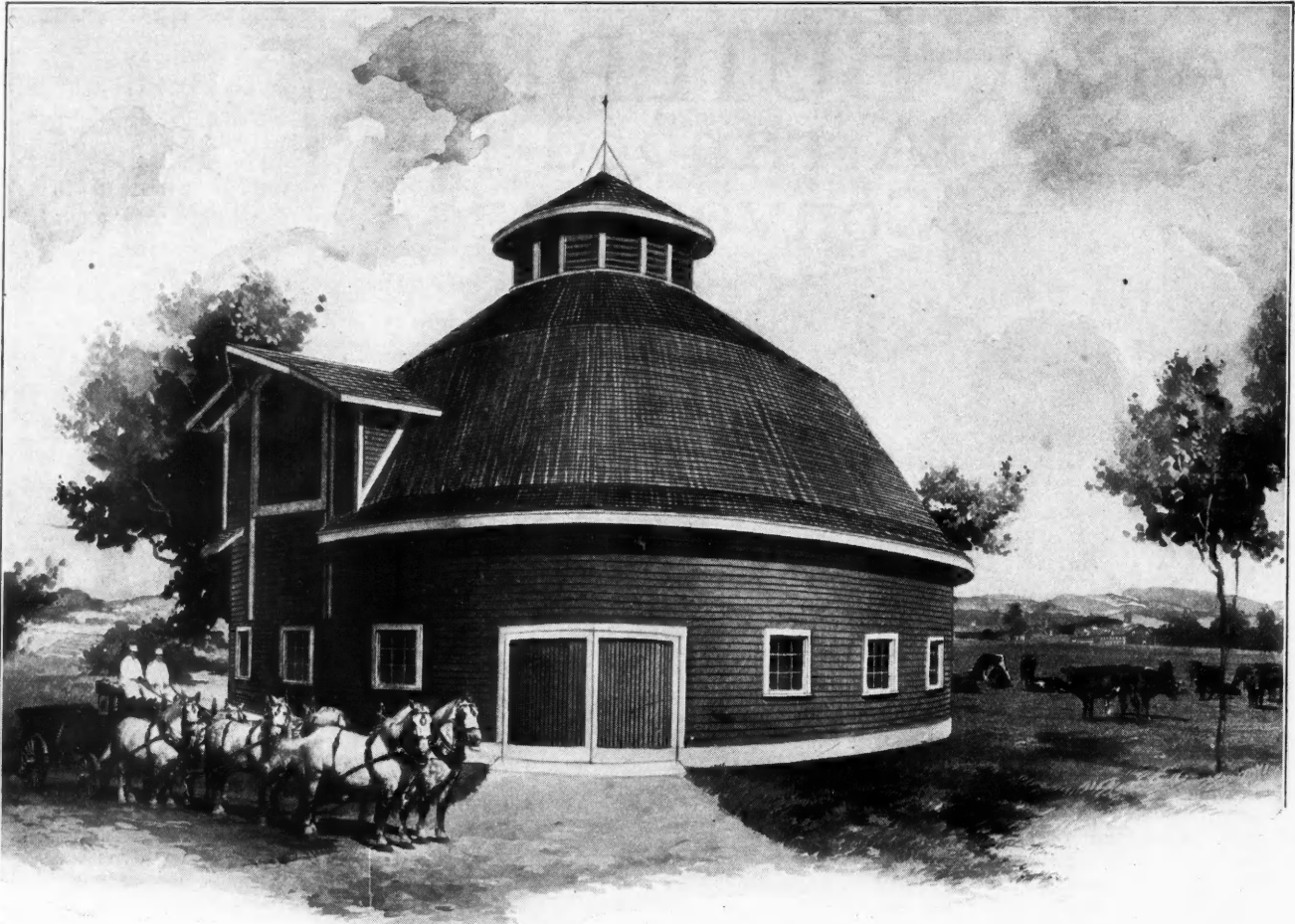
Sixty-foot round barn arranged one-half for horses and one-half for cows. A 14-foot silo occupies the center and a gable end dormer gives access to the big circular hay mow. We can furnish complete set of blue printed working plans and typewritten specifications for only $12.00 per set. When ordering, ask for Design No. A305.
