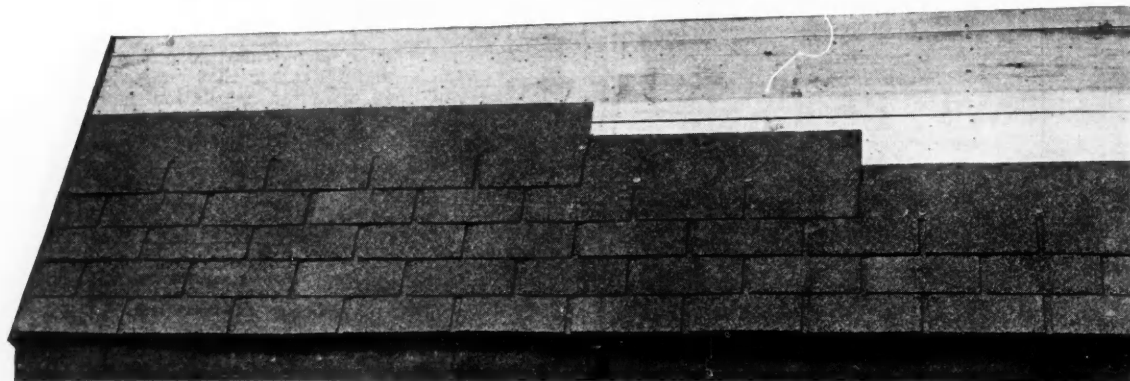
"Rex" Strip Shingles Measure 40 by 10 inches—Five Shingles to the Strip.
