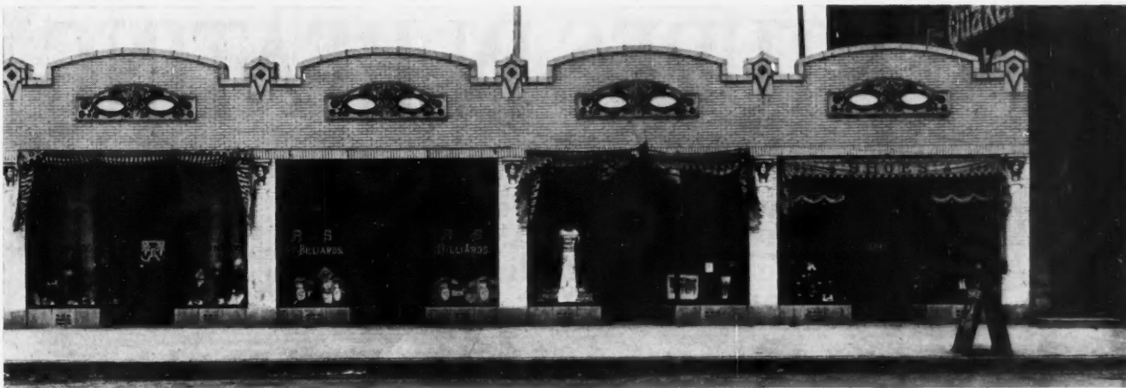
One-Story Group of Stores Combining Ornamental Terra Cotta and White Enameled Brick in a Very Decorative Design.
