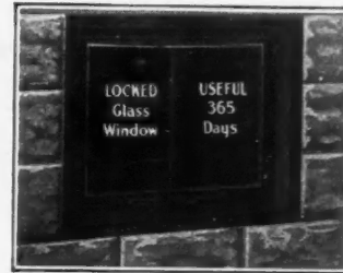
A Light Basement
