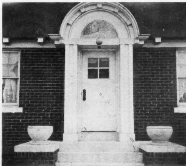
A Pictorial Cement Slab over Doorway.
