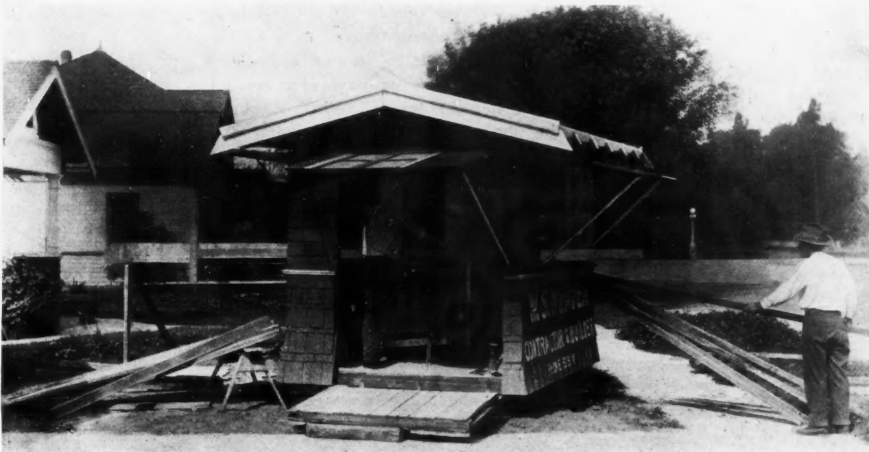
PORTABLE WOODWORKING SHOP FOR BUNGALOW BUILDING.
