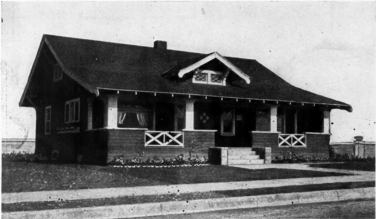
A Typical California Bungalow Design. It is 44 by 29 feet in size, having five rooms and a bath room, with a good cellar and a stairway to the attic. We can furnish complete set of blue-printed working plans and typewritten specifications for only $7.00 per set. Blue-prints consist of basement plan; roof plan; first and second floor plans; front, rear, two side elevations; wall sections; and all necessary interior details. Specifications consist of twenty-two pages of typewritten matter. When ordering, ask for Design No. 6607.
