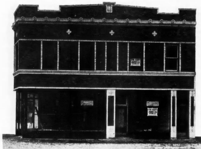
A. P. Gassmann & Co., Architects (Construction Photograph)
