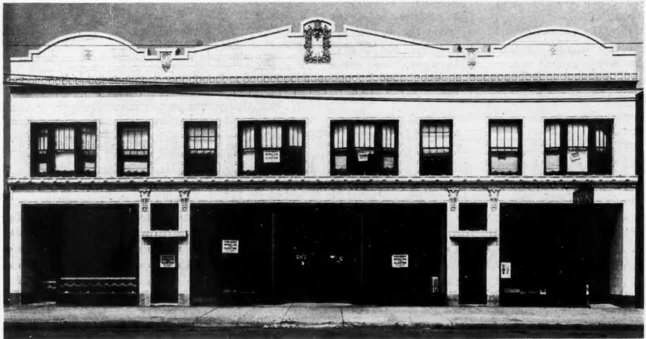
Group of Three Stores on an Inside Lot; a Two-Story Building; Front is Entirely White Enameled Terra Cotta; a Combination of Plain and Ornamental Pieces.
