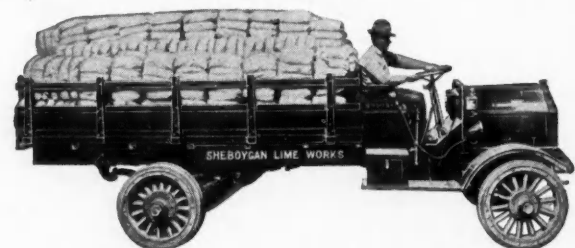
KisselKar Truck in Service of Sheboygan Lime Works
