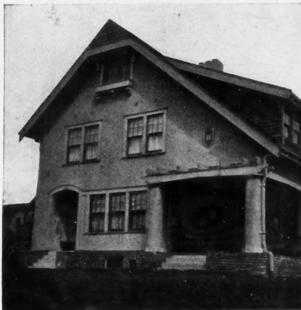
Slab of Cement Bearing an Ornamental Colored Design Inset over Porch.
