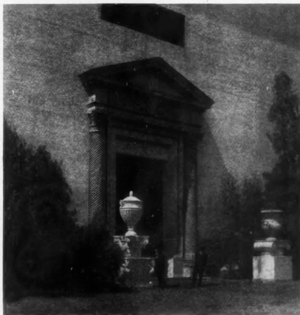
One of the south entrances of the Palace of Education. The exterior finish of the Exposition buildings is in imitation Travertine marble and the old ivory shade of this material is the key color of the buildings and grounds. The composition used in this exterior finishing is a specially prepared gypsum product.
