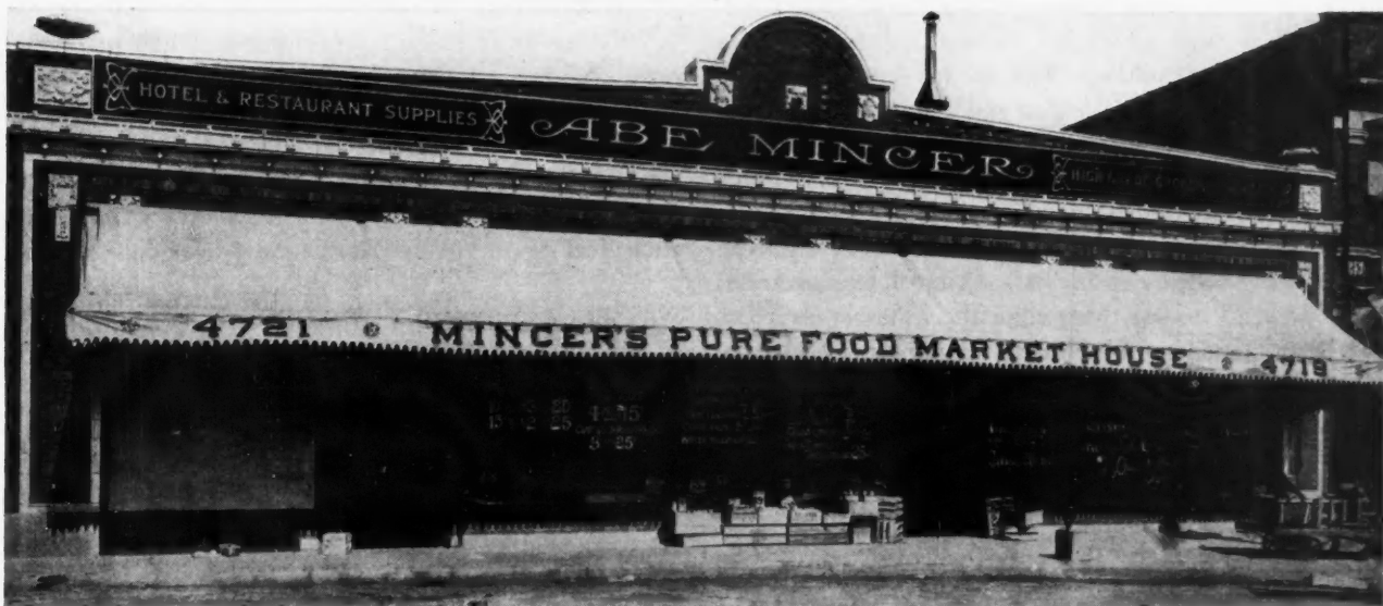
An Attractive Business Place—One-Story High on an Inside Lot; Front Composed of Dark Rough Texture Brick with White Enameled Terra Cotta Trim.
