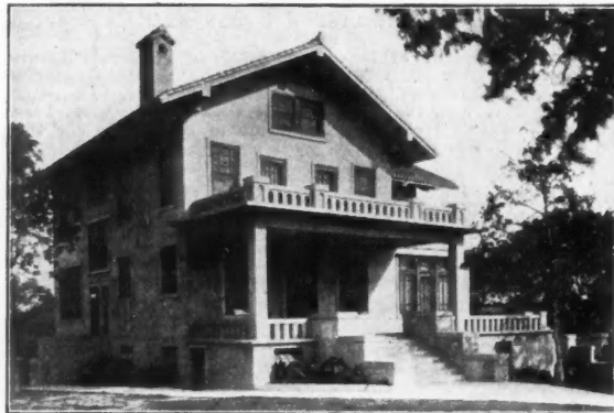
Residence of C. A. Mangold, Oak Cliff, Dallas, Tex. Stucco on RIB LATH.
