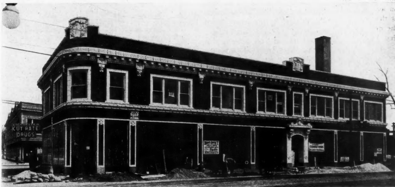
A Corner Business Block Two-Stories High; Constructed of Brown Vitrified Brick and White Enameled Terra Cotta Trim. Photograph Taken During Construction.
