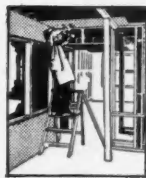
Method of supporting ceiling panels
