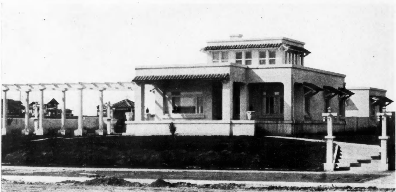
Home of Louis Purcell, of Long Beach, Cal., built at Los Cerritos, a suburb of that city. Built of reinforced concrete throughout.
