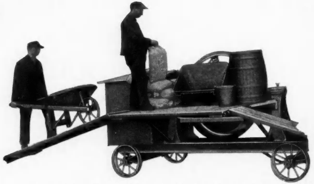
Clover Leaf Mixer with Handy Side Loading Platform.
