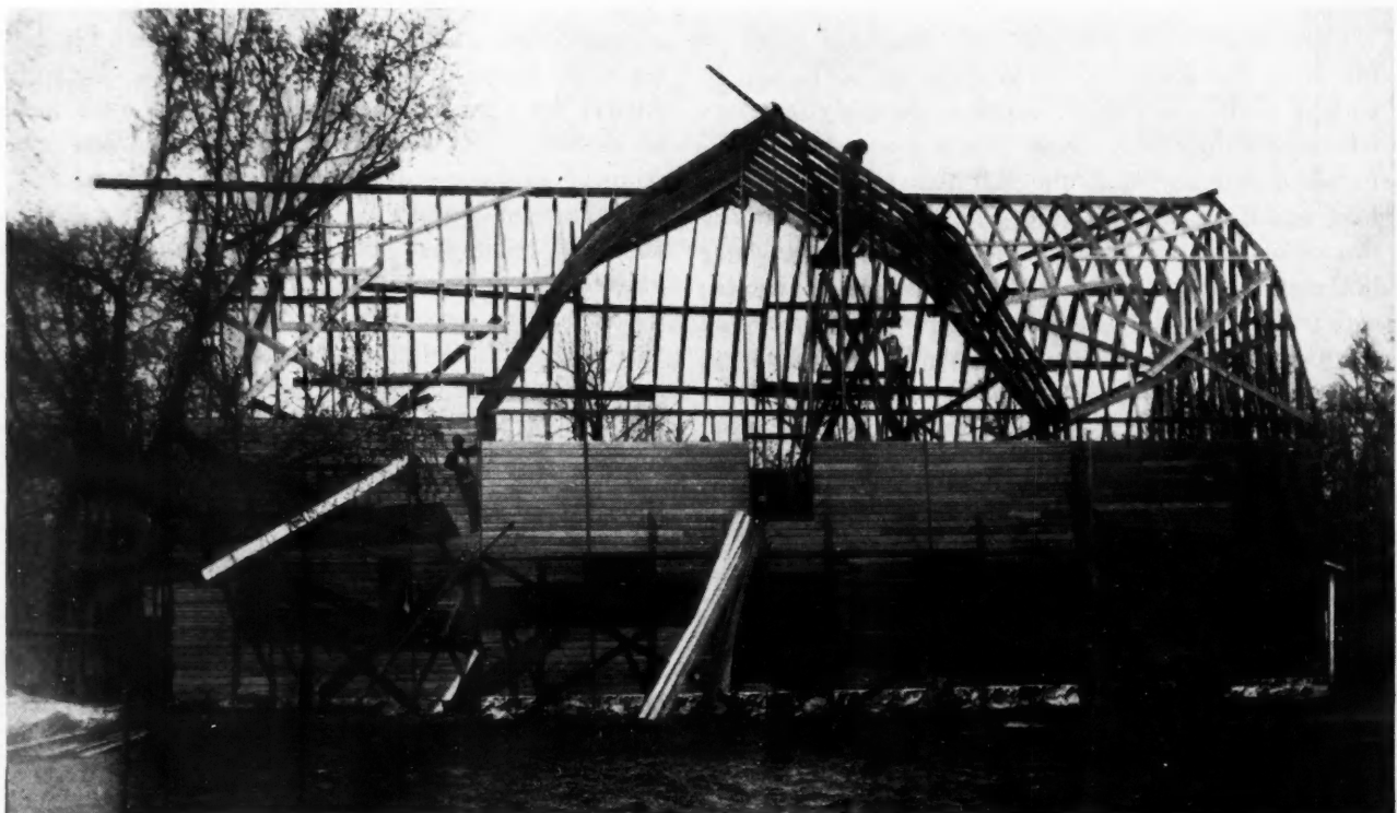
View of Barn During Construction—Note Right-Angle Gambrel Roof Framing.
