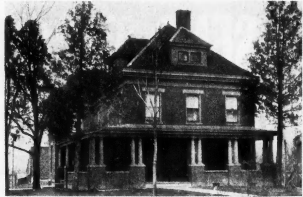
Fine Residence of Fred Huggins, Crawfordsville, Ind., Lighted with Johnson System.
