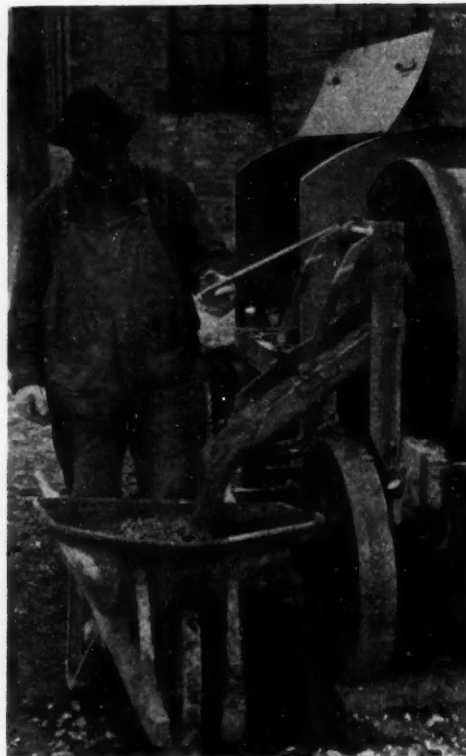
"Atlas" Mixer Is Easily Dumped.
