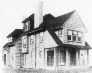
Residence of F. L. Grant, Shaker Heights, Cleveland. Architect, Mr. Wm. Powell. Gray Shingles on Side Walls; Darker Shade on Roof.
