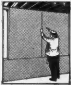
Nail edges with flat-head nails.
