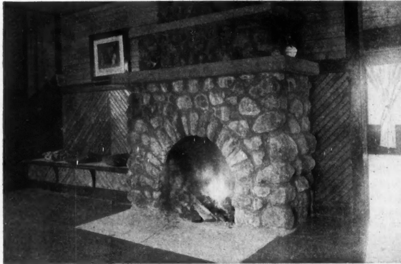
Rough Cobblestone Fireplace Built with Self-Supporting Stone Arch, in Summer Cottage of Minford Backus, at Star Lake, N. Y.
