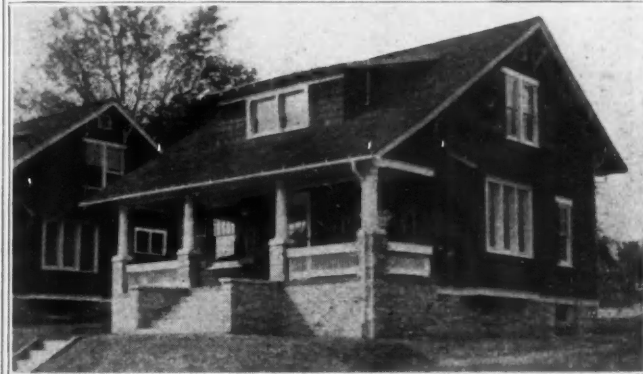
Birch-finished, 6-room Bungalow at Hyattsville, Md. Stone foundation and fireplace, tiled bathroom, beamed ceilings. Chas. M. Lightbown, builder.
