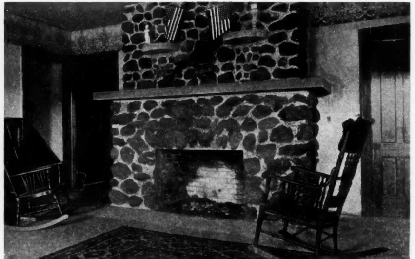
Neatly Finished Cobblestone Fireplace and Chimney. Each Stone Abounds With Color
