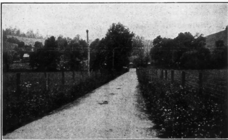
Twelve-Foot Concrete Road at Whitehall, Md. This is the Type of Road that Has Proved to be a Veritable Boon to the Farmers. It is an Ideal Thoroughfare to Walk Upon as Well as a Road, Never Accumulating Mud or Dust
