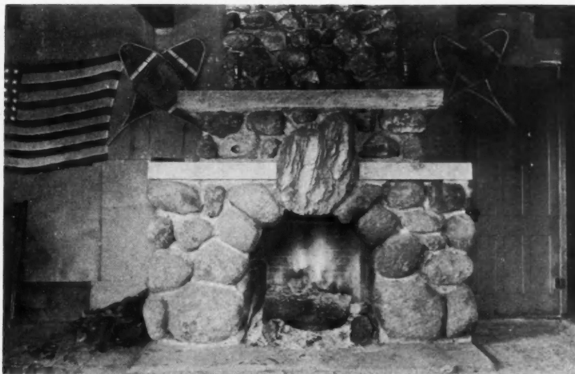
Unique Stone Fireplace in the Summer Home of James Whittington, Star Lake, New York. Large, Undressed Stones Form the Arch and Smaller Stones the Chimney. Mantel Shelves are Concrete Slabs
