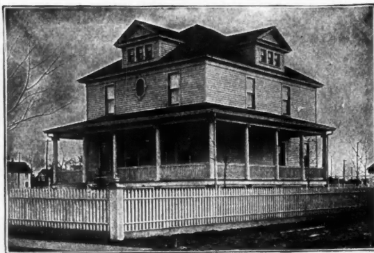
Residence of Jos. Bagnarello, Freeport, N. Y. Entire cellar waterproofed successfully against 1-foot water pressure by the use of Ceresit. A. S. Johnson, Contractor.
