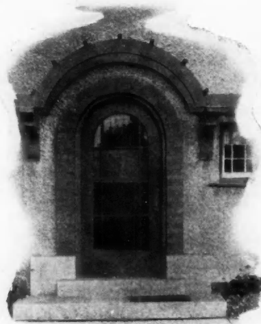
Simple entrance doorway finished with brick. They are arranging entrances like this on the side, leaving the entire front of the modern home for screened living porch.
