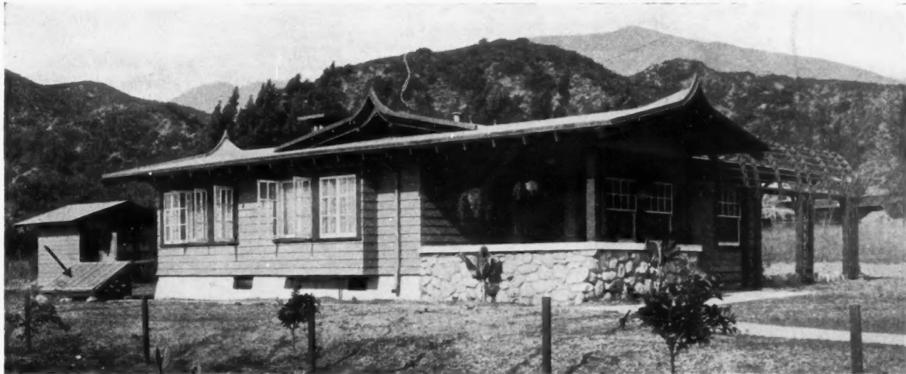
California Bungalow with Sun Coil near Ground at Rear of Building
