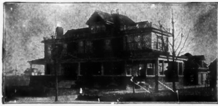
Residence of Thos. Forbes, Freeport, N. Y. Cellar floor subject to 2-foot water pressure. Furnace pit subject to 3-foot water pressure. Entire cellar, about 1500 sq. ft., waterproofed thoroughly by the use of Ceresit. A. S. Johnson, Freeport, Contractor.
