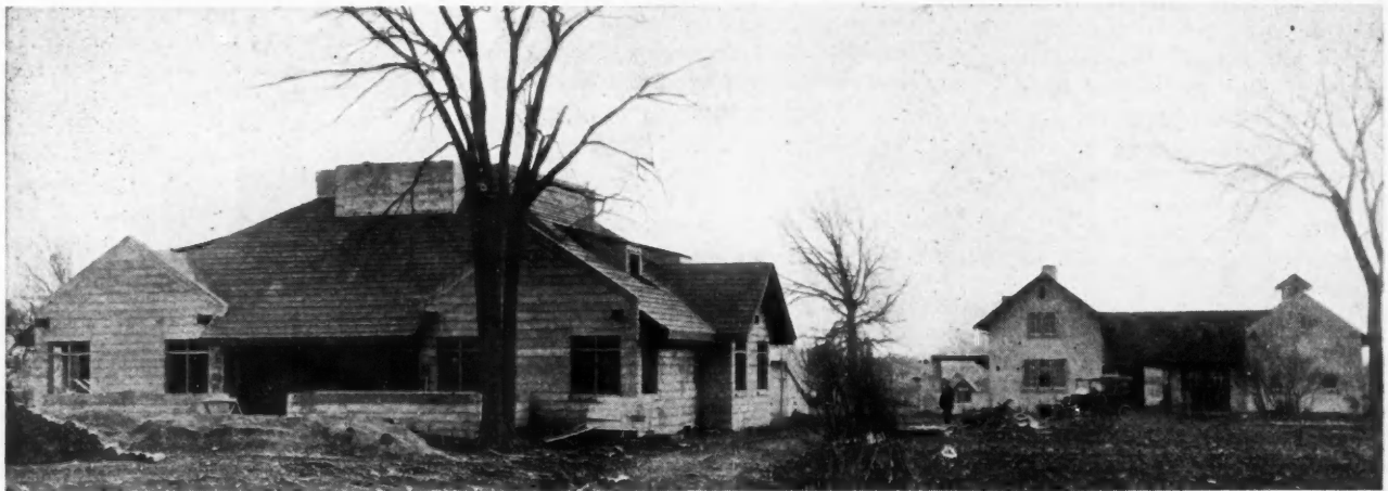
Residence Country-Place Structures of Dr. Charles R. Pullen, Rochester, N. Y., Built with Double Concrete Walls Cottage, Garage, Stable
