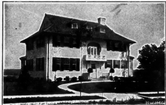
Residence of John Neuscheler, River Edge, N. J. Wilder & White, Architects Covered with J-M Asbestos stucco
