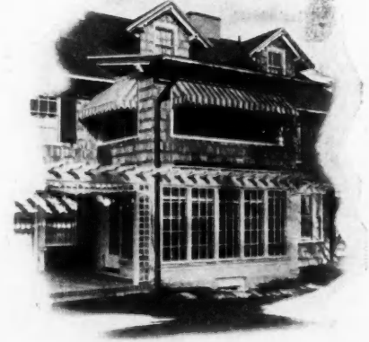
Well designed two-story porch on a shingled house. First floor is sun parlor and second floor balcony or sleeping porch.
