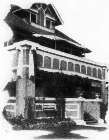
Rough finished cement plaster with ornamental wood paneling is being much used. The lintel of this broad porch is well trussed to prevent sagging.
