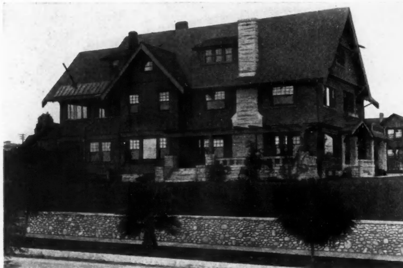
Fine Residence of F. D. Butterfield, Los Angeles, Who Writes That for Two Years the Solar Heater on the Roof Has Furnished Hot Water for Three Bath Rooms in This House. The Ruud Heater Connected Up with It is Seldom Needed.
