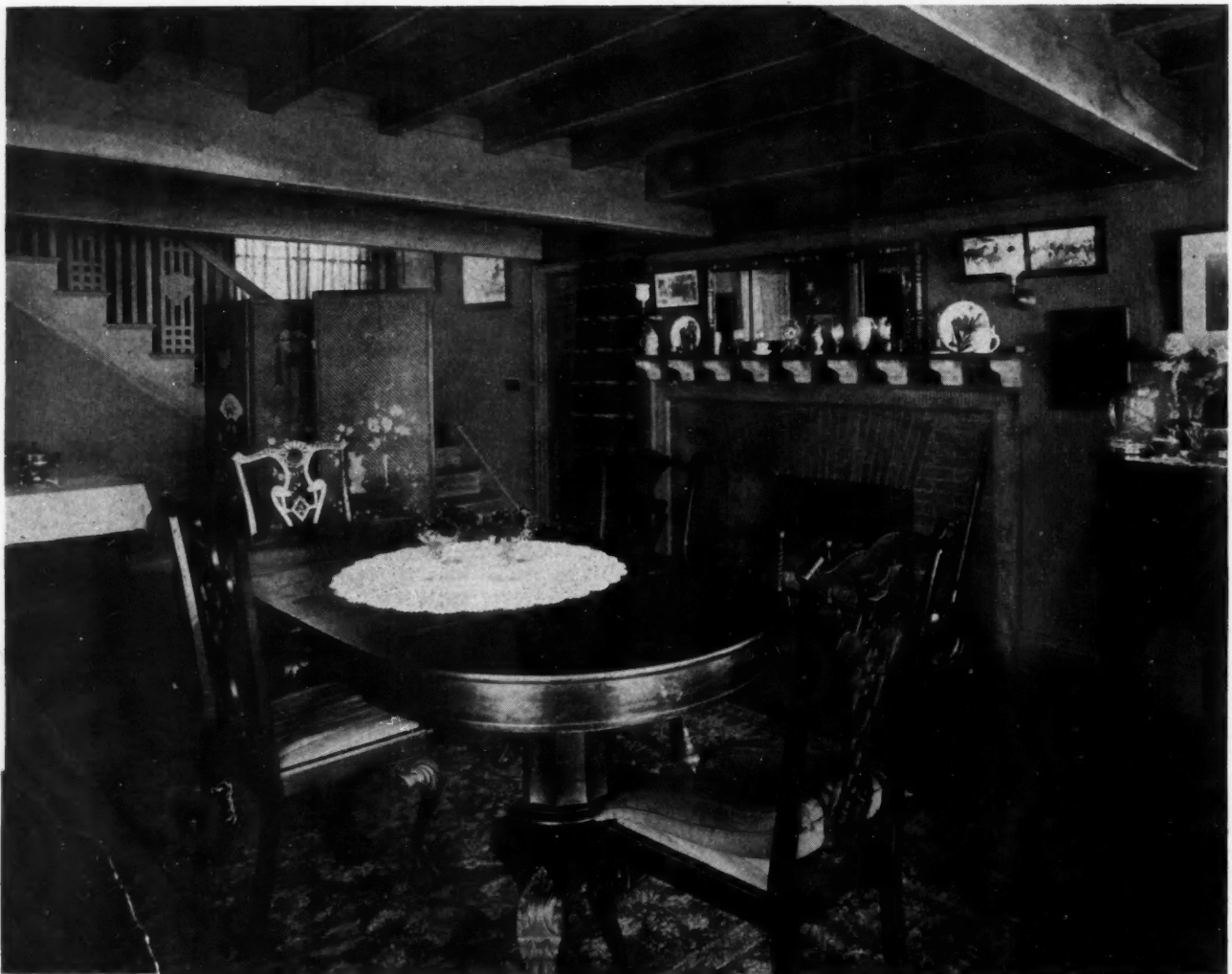
Remodelled interior of old New England homestead, showing genuine heavy oak ceiling beams. These carry the weight of the floor above. Modern beams are tacked on for ornamental effect. They carry no weight.
