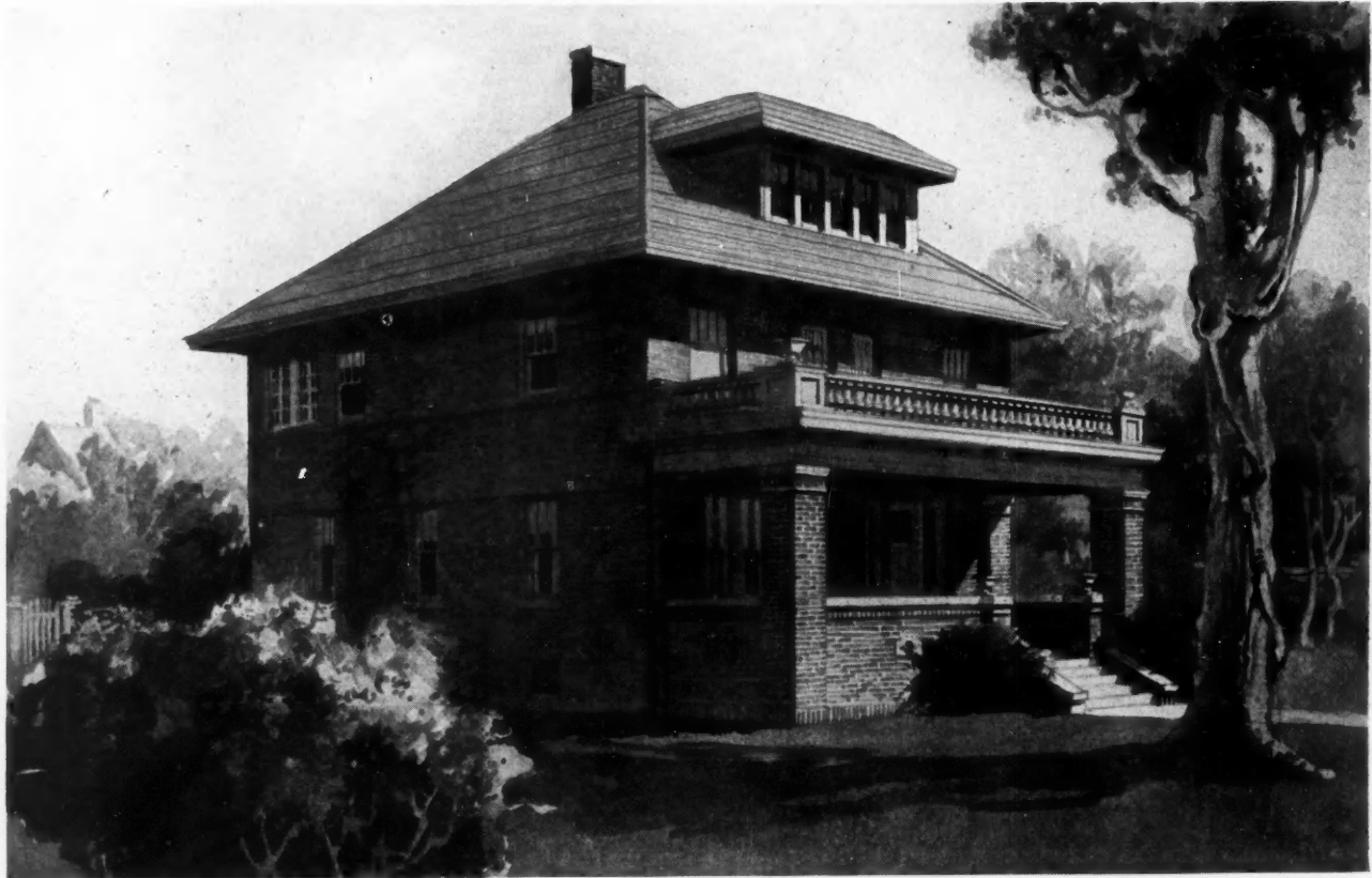
Rich eight-room brick residence. Size 31 by 34 feet 6 inches. A popular hip-roof design. We can furnish complete set of blue-printed working plans and typewritten specifications for only $15.00 per set. Blue prints consist of basement plan; roof plan; first and second floor plans; front, rear, two side elevations; wall sections and all necessary interior details. Specifications consist of twenty-two pages of typewritten matter. Ask for Design No. 6543.
