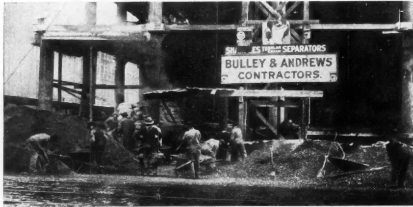
Fig. 3. Sand and Gravel Heated by Steam
