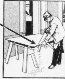
SAWING Use a fine, panel saw, as for any fine lumber, pebbled side of panel up.
