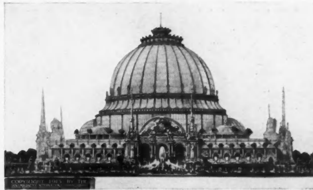
Horticultural Building, which will be 630 by 295 feet—one of the most notable structures of the kind ever built, being composed almost entirely of glass; set in the west end of the south garden opposite the Palace of Education, its glittering dome, 165 feet high, will be seen as one of the striking features of the exposition.
