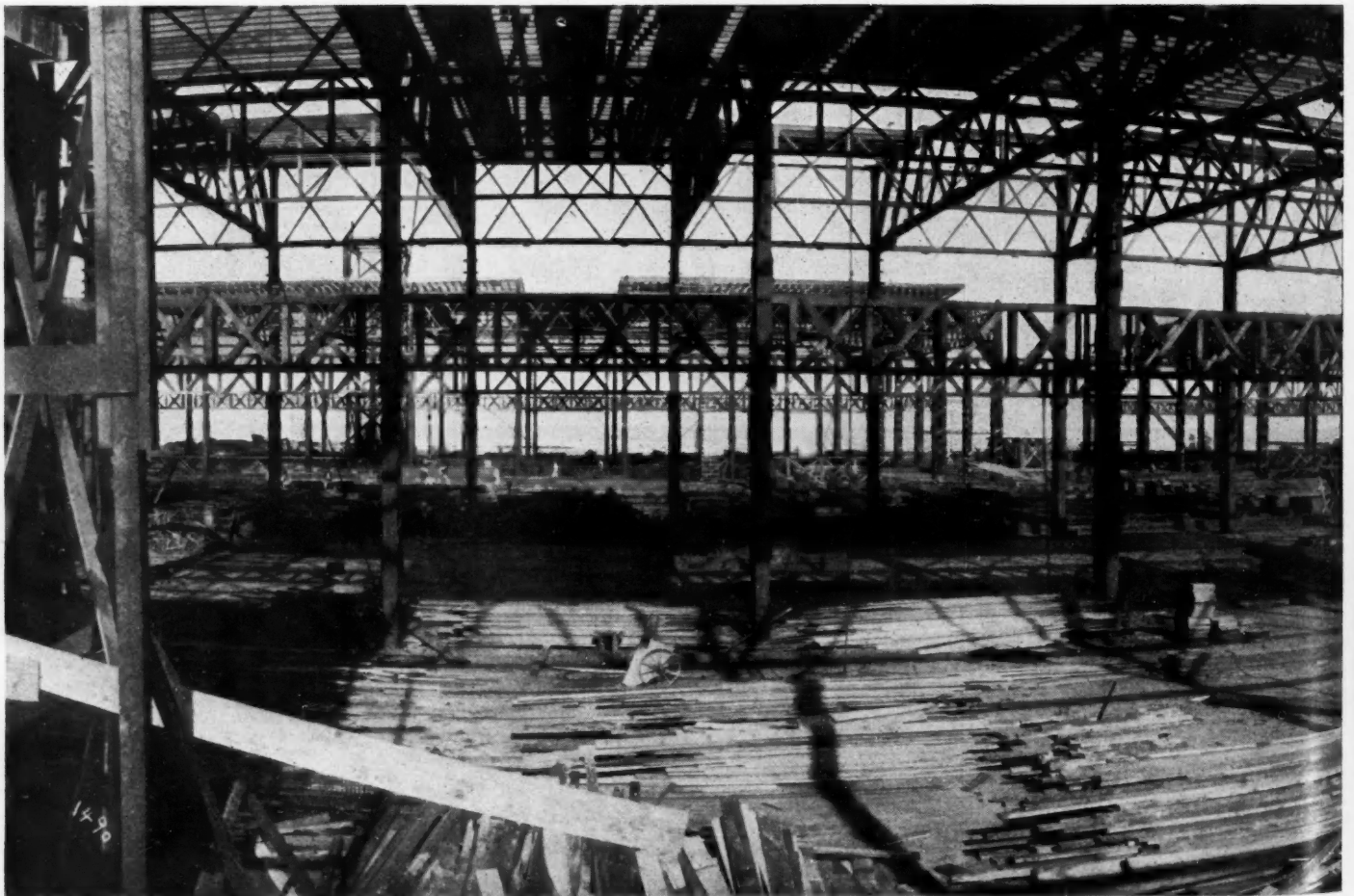
The Palace of Food Products, one of the main exhibit palaces of the Panama-Pacific International Exposition, as it now appears. 45 per cent completed. Upon that date, 900,000 feet of material had been placed and used in the construction. Compared with the already completed Palace of Machinery, the largest wooden building the world has ever employed to ensure the finishing of the exposition on time. The Palace of Food Products covers ground to the top of the dome
