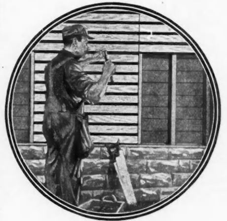
Keyed Lath Keeps Plaster In and Up
