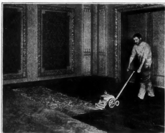
Old Varnished Floor Being Easily Refinished With Machine
