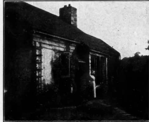
Home of J. Acker Hayes—Stucco Stained with Cabot's
