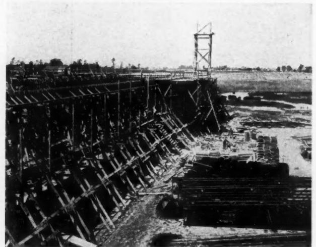
Form Work on New Beaver Board Plant at Thorold, Ont.
