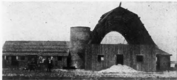
Large Barn Being Built by W. A. Richter
