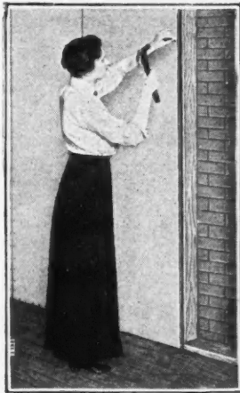
Applying Direct to Studding
