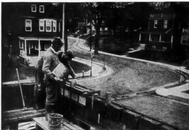
Making ready to insert the floor beams.
