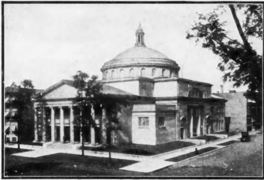
Asbestos "Century" Shingle Roof — Eighth Church of Christ, Scientist — Michigan Avenue and Forty-Fourth Street, Chicago, Ill. — Architect, L. E. Stanhope, Chicago, Ill.
