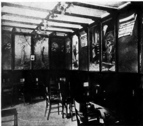
Grill Room in Goetz Bros' Restaurant, New York City—Hand Painted Panels
