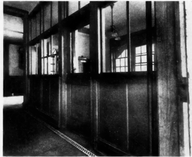
Entrance to the Wm. Cramp & Sons Ship and Engine Building Co. Phila. Pa. Where the Compo-Board joins is covered by a half-inch round Moulding
