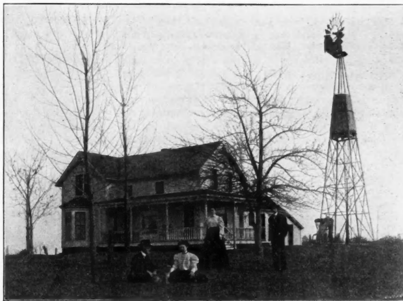
Farm Residence of Mr. Theodore Hartsell, Eau Claire, Mich., Lighted by Davis Acetylene Lighting Plant. More than 300 other farm homes within a radius of 30 miles of this home are equipped with Davis lighting outfits.
