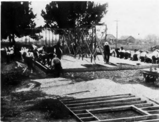
9:30 A. M., Wall Framing Being Raised
