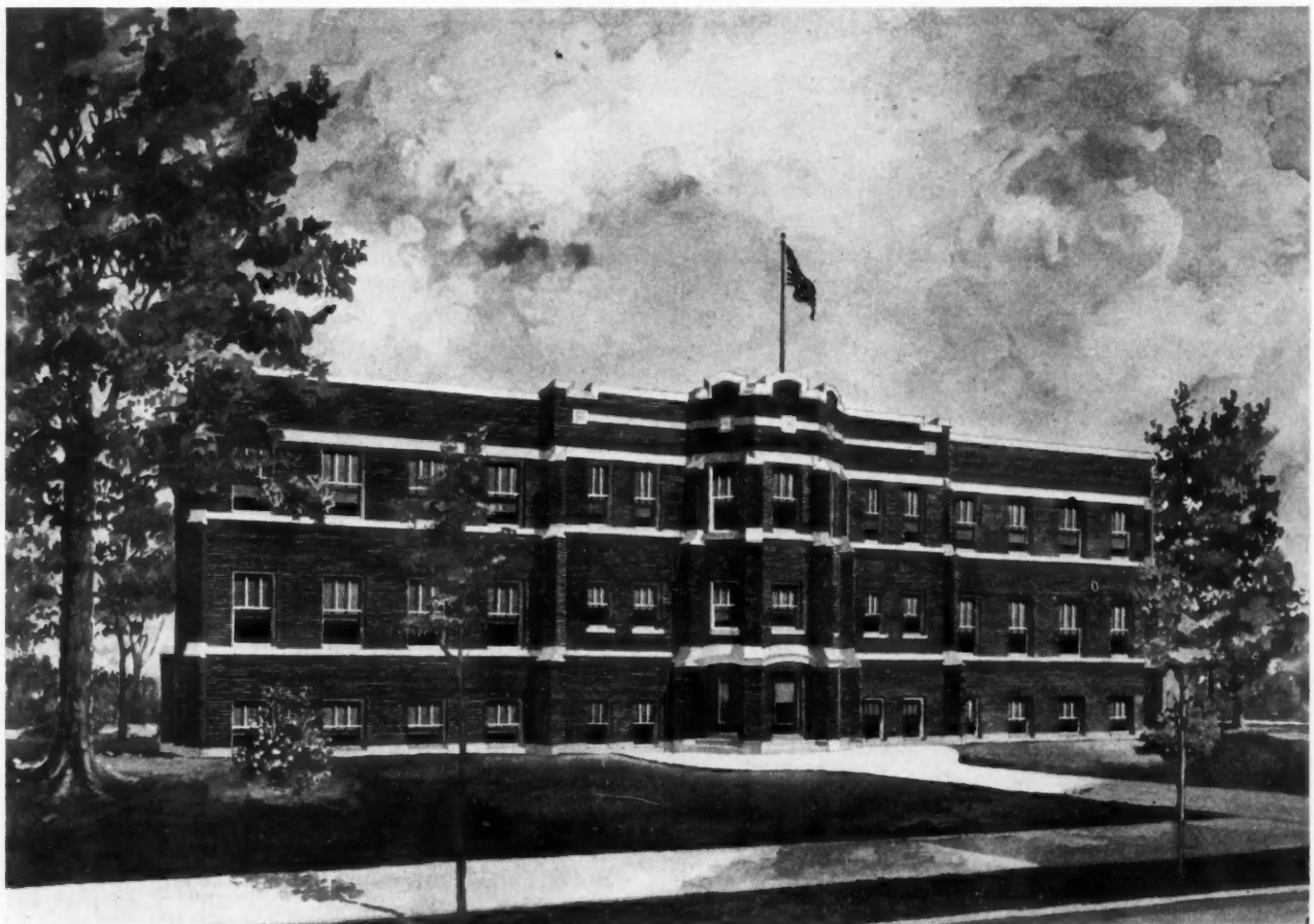
Up-to-Date Public School Building with Facilities for Neighborhood Meetings, Etc.
