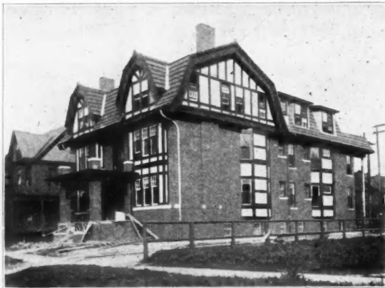
Mineral Surfaced Ready Roofing Used as Siding on the Upper Story and in the Panels of the Bay Windows—New Detroit Apartment Building
