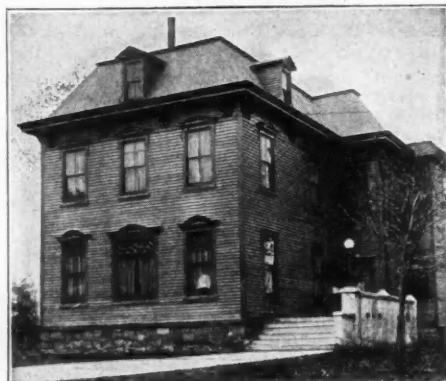
MARQUETTE CLUB, Marquette, Michigan Roofed with "BURMITE."
