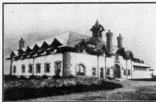
Asbestos "Century" Shingle Roof—Stable of Theodore M. Davis, Newport, R. I.; Theodore Davis Boal, Washington, D. C., Architect; Simpson Bros. Corp., Boston, Mass., Contractor
