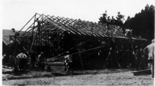
10:30 A., M. Rafters in Place
