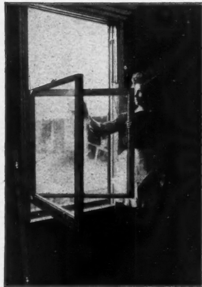
Both Sashes Swung into Building
