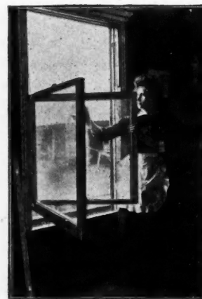
Both Sashes Swung Into Building
