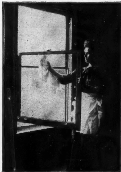
Lower Sash Swung into Building
