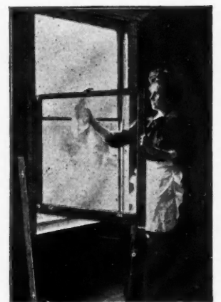
Lower Sash Swung Into Building
