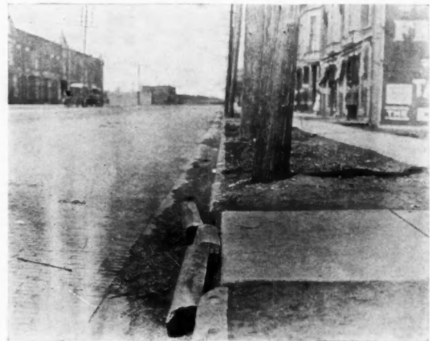
Result of Building Curb Next to Walk
