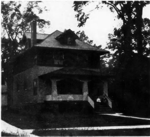
A Typical Suburban Home
