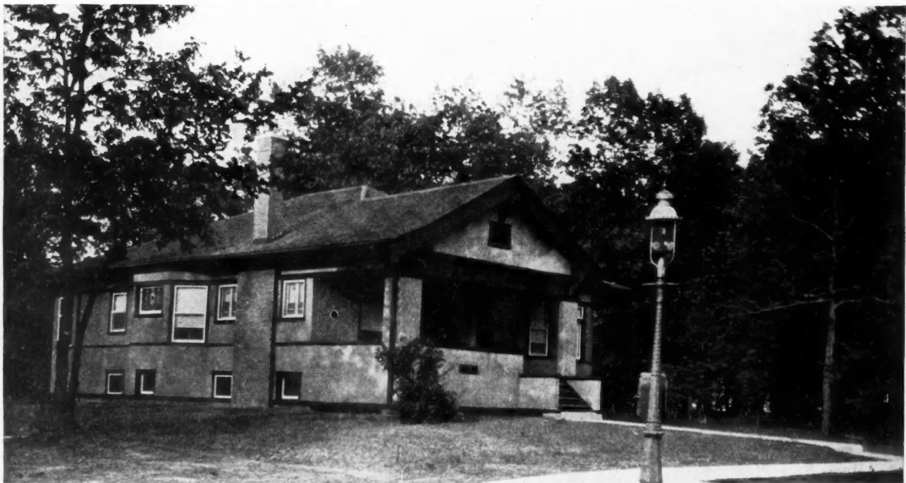
Large Well-Shaded Lots Make the Bungalow Type of House Especially Attractive
