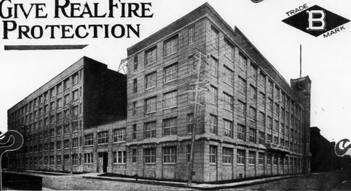
The New Keuffel & Esser Building, Hoboken, Covered with Barrett Specification Roof
