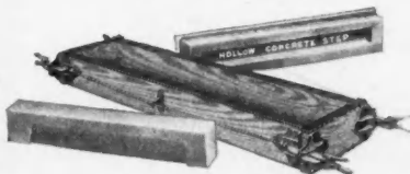
Ideal Cement Sill Mold
