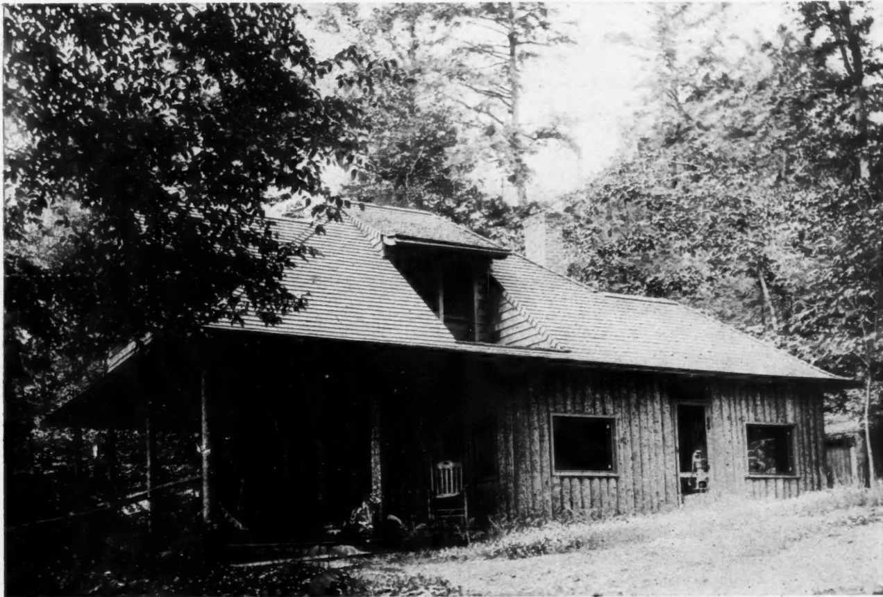
Slab and Shingle Construction
