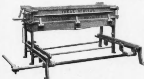
Ideal Special Sill and Lintel Machine
