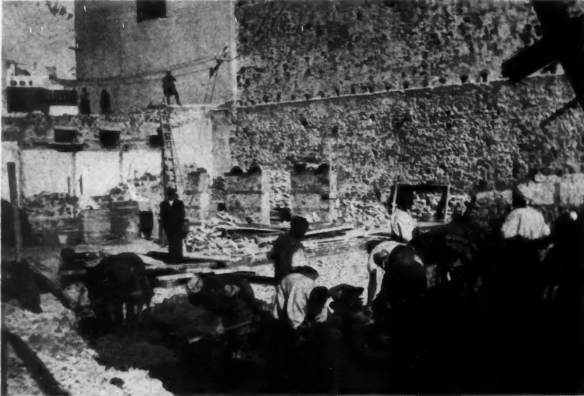
Excavating for a Building
