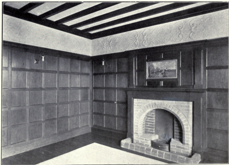
The Hatch Heath, Beds, J. T. LAWRENCE, Architect. Oak Panelling ; THE FORWARD CABINET WORKS, Wealdstone, Middlesex.
