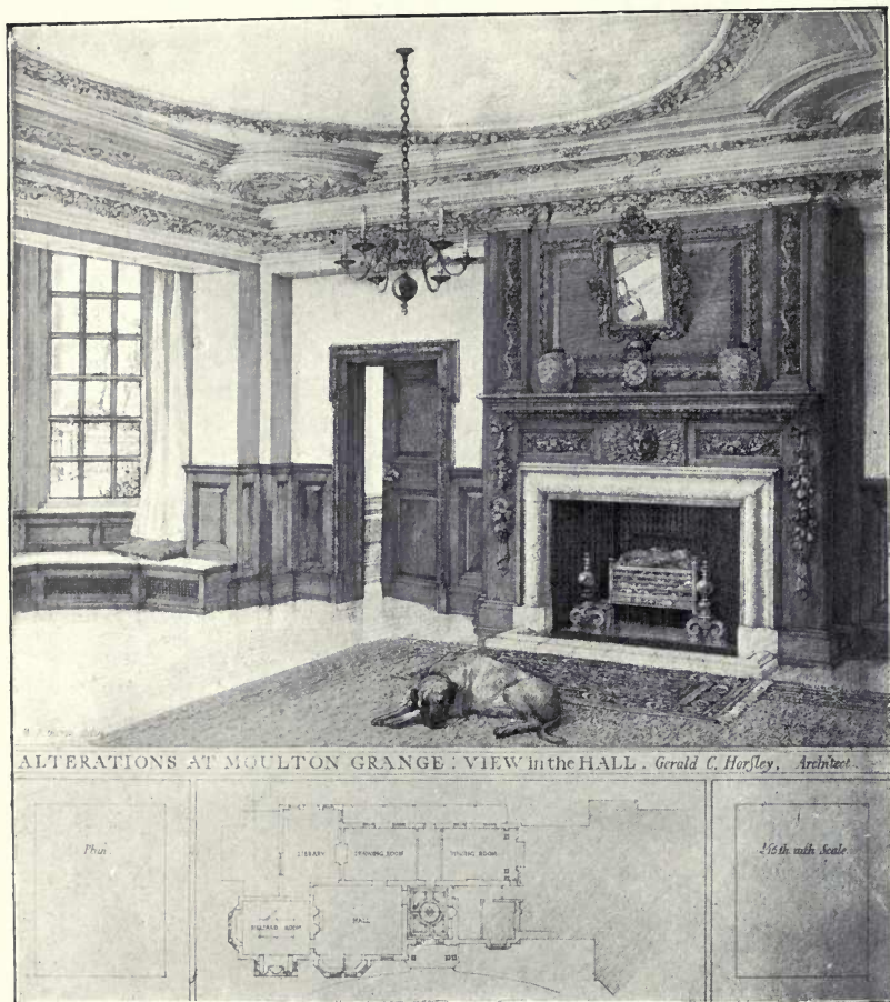
Alterations at Moulton Grange, GERALD C. HORSLEY, Architect.
