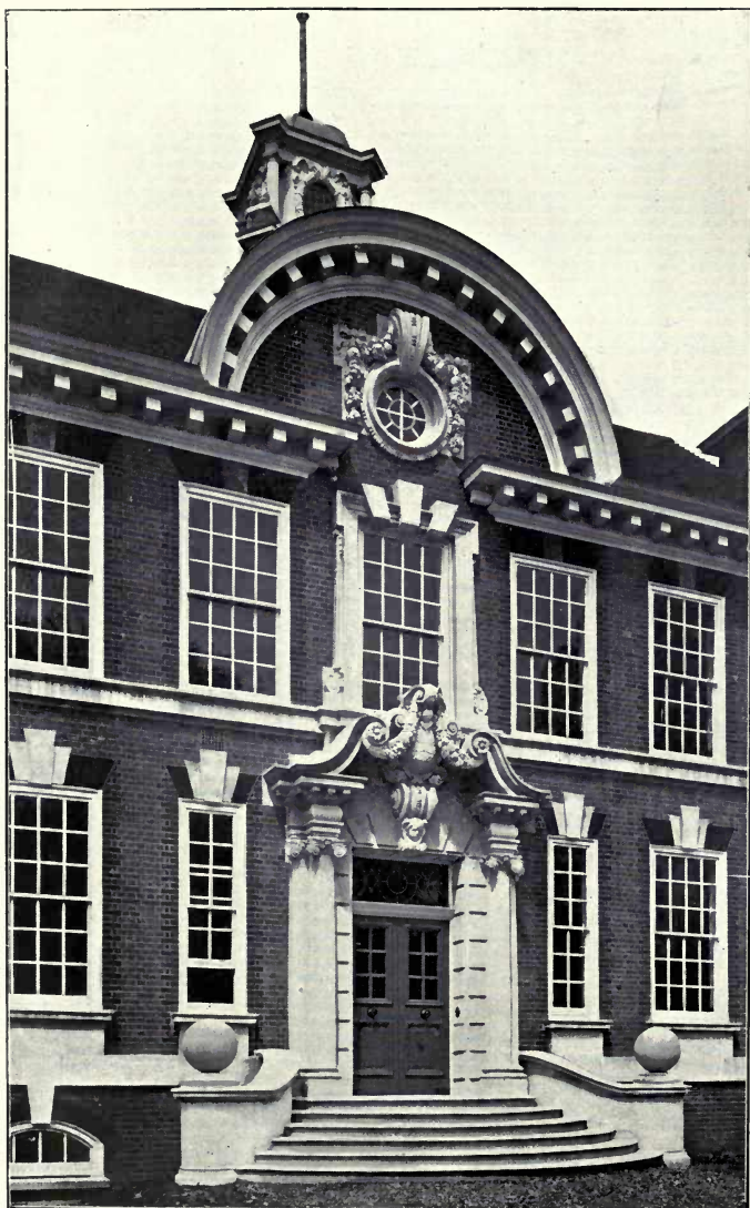
Main Entrance, The New County School for Boys, Bromley, Kent, H. P. BURKE DOWNING, Architect.
