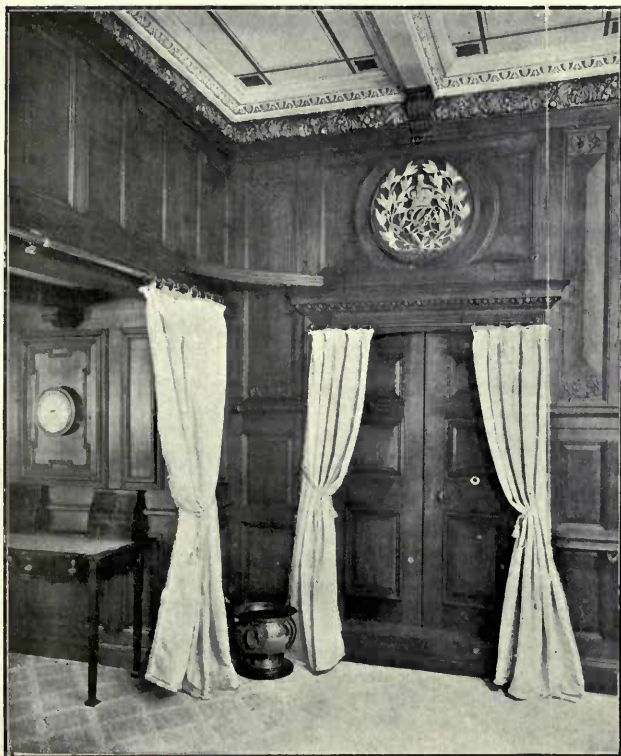
Entrance to Royal Apartments, S.S. "Medina." T. E. COLLCUTT, Architect.
