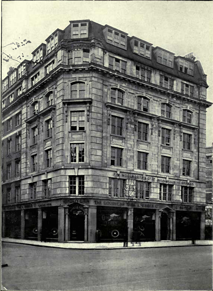
Central House, Kingsway, TREHEARNE & NORMAN, Architects.
