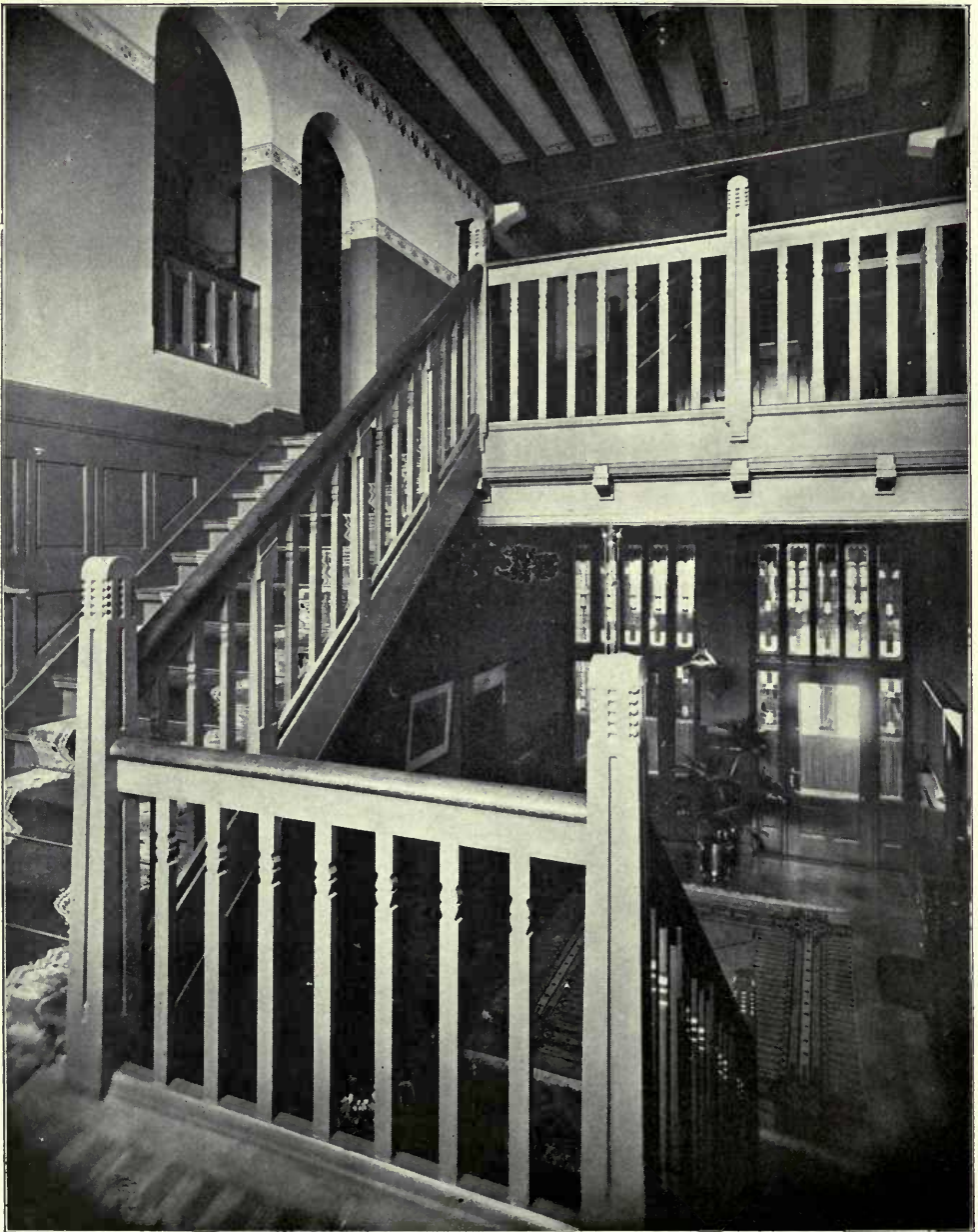
Staircase, ED. CUYPERS, Architect.
