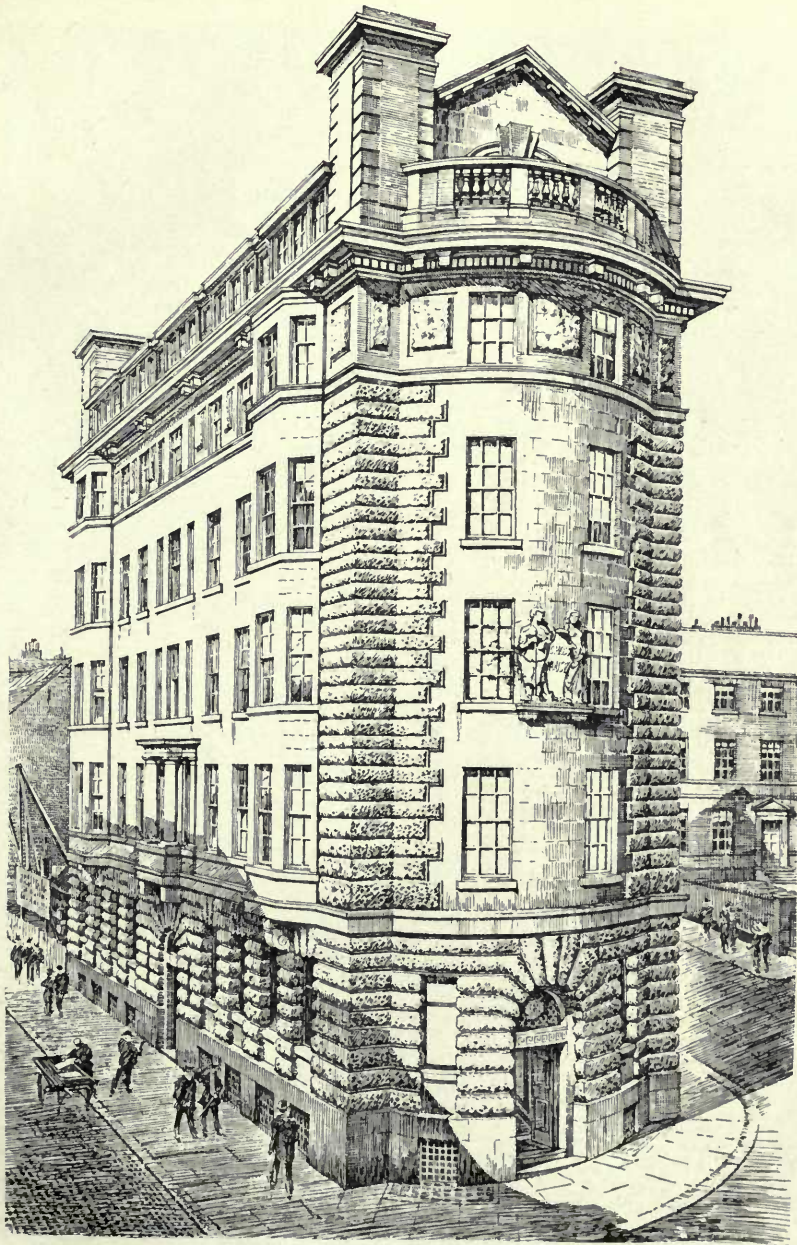
Cross House, Newcastle-on-Tyne, CACKETT & DICK, Architects. Heating and Ventilating and Hot Water Supply, WALTER DIX & Co., Low Bridge, Newcastle-on-Tyne.
