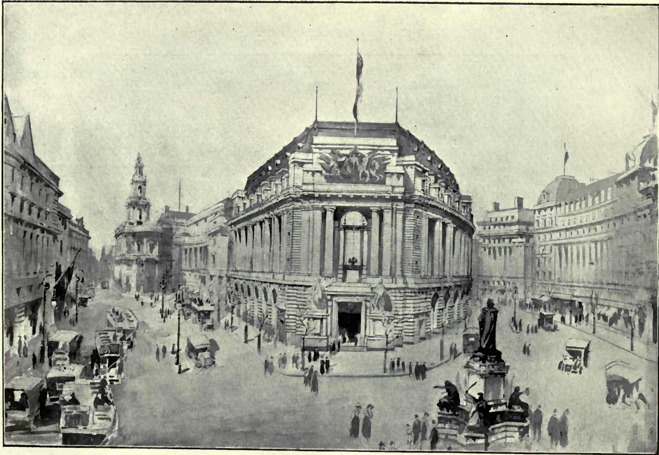
The Commonwealth Building, London, W.C., A. MARSHALL AND A. G. R. MACKENZIE, Architects.
