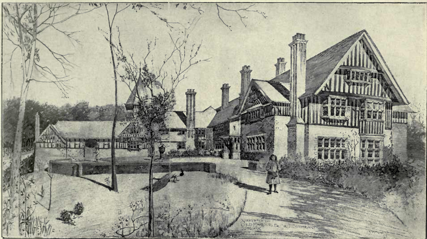
Liphook, Residence for Sir Thomas Sutherland, T. E. COLLCUTT, Architect.
