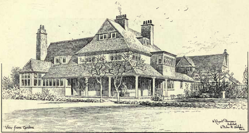
1454. Bronygarth, Woldingham, W. RUPERT DAVISON, Architect.
