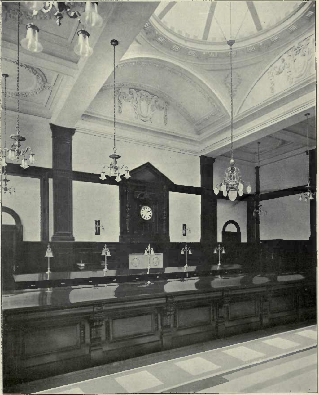
357. Glasgow Savings Bank, Parkhead Branch , HONEYMAN, KEPPIE AND MACKINTOSH, Architects. (For Plans, see p. 92.)
