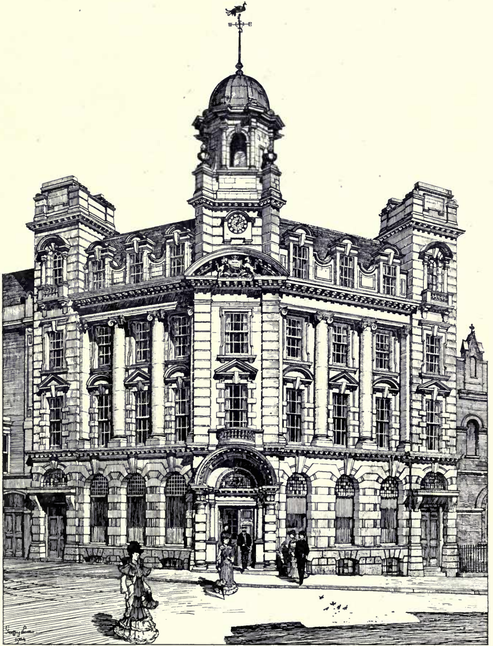
New Buildings, North Street, Brighton, for the Royal Insurance Co., CLAYTON AND BLACK, Architects. Mosaic Floors: The Art Pavements and Decorations, Ltd., 7 Emerald Street, Theobalds Road, London, W.C. General Contractors: W. A. Field and Co., 20 Preston Street, Brighton.
