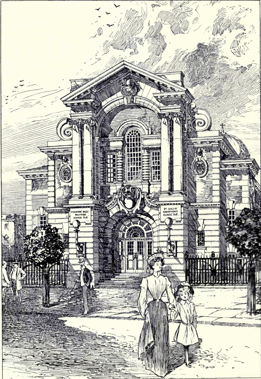
1617. West Front of a New Church at Peckham, H. P. BURKE DOWNING, Architect.
