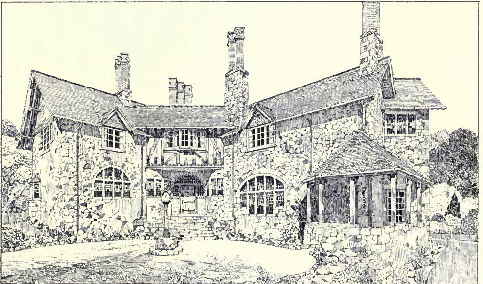
1487. House at Garn Hill, St. Andrews, near Cardiff , J. COATES CARTER, Architect. (For Plans, see p. 48.)
