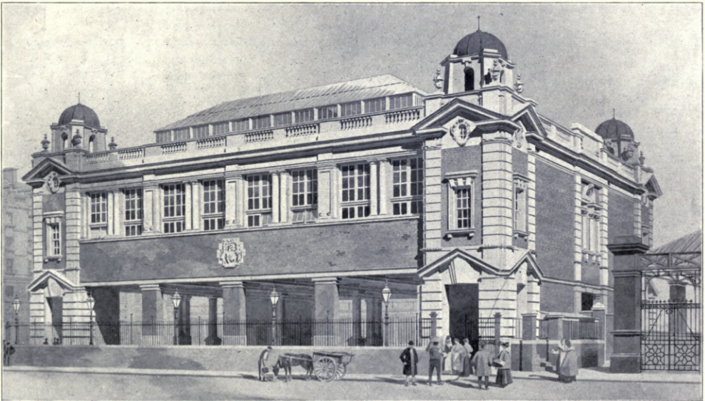
1459. New Foreign Flower Market, Covent Garden, W.C. , LANDER, BEDELLS AND CROMPTON, Architects. Contractors for Superstructure: Howard and Co., Broad Court, Bow Street, London, W.C.
