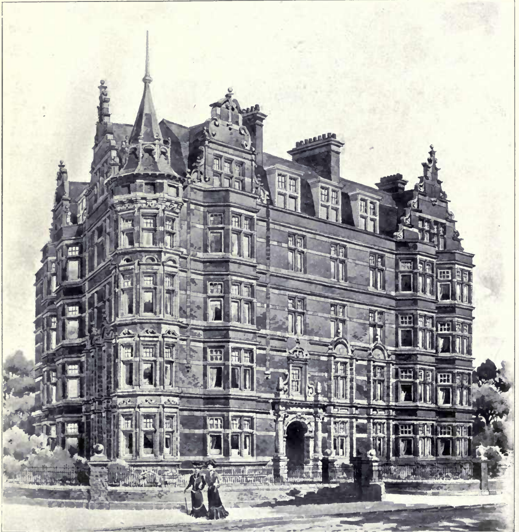
Albemarle Mansions, Hampstead, N.W., JAMES F. C. BELL, Architect. W. J. King, Builder and Contractor, Hampstead, London, N.W. Constructional Steel and Ornamental Wrought Iron Work, B. Bridgwater and Co., Ltd., 78 York Road, King's Cross, N. (For Plan, see p. 115.)
