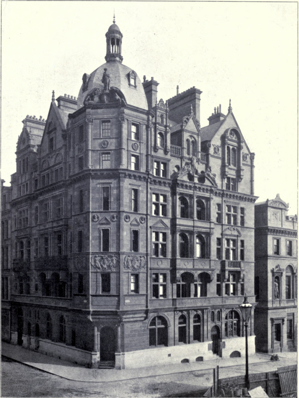
440. The Offices of the Sun Insurance Co., Glasgow, WILLIAM LEIPER, R.S.A., Architect.
