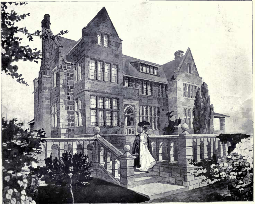
Residence for Capt. Frederick M. Alger, at Grosse Pointe Farms, Mich., STRATTON AND BALDWIN, Architects. (For Plans, see p. 87.)
