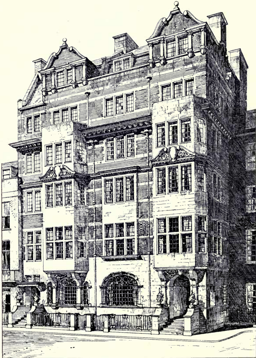
1534. Nos. 10 and 11 Park Place, St. James', S.W., HART AND WATERHOUSE, Architects.
