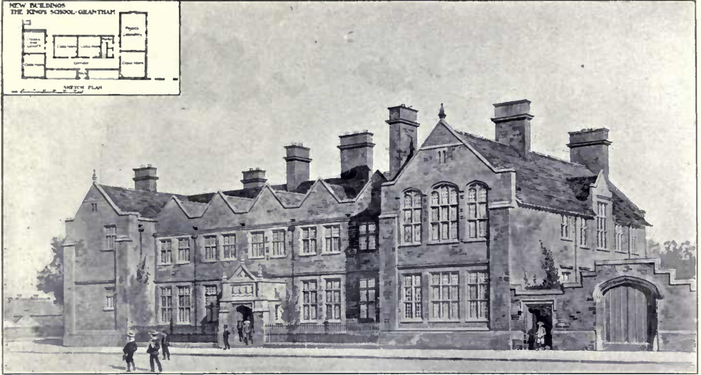
1581. Grantham Grammar School , JOHN BILSON, Architect. General Contractors: Hockley and Co., Grantham.
