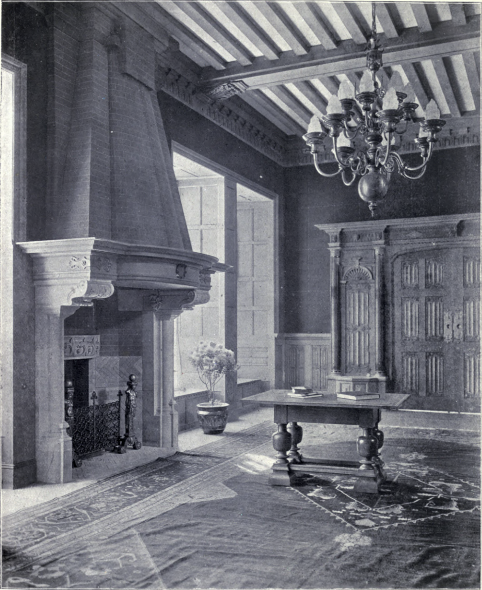
417. The Hall, Parkwood, Henley-on-Thames, WILLIAM FLOCKHART, Architect. Executed by J. S. HENRY.
