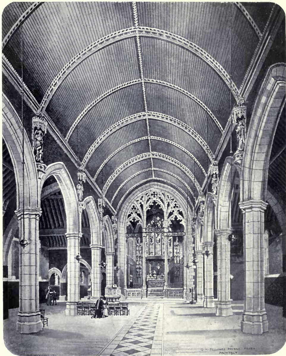
1583. New Church, Belvedere, Kent, Interior View, looking East , G. H. FELLOWES PRYNNE, Architect.
