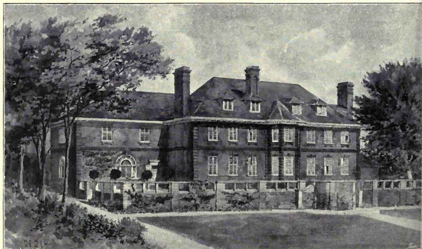
1790. Frithwood House, Northwood , MERVYN E. MACARTNEY, Architect. (For Plans, see p. 29.)
