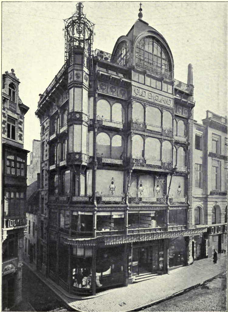
Magasin Old England, Brussels, PAUL SAINTENOÏ, Architect, Brussels. (In collaboration with MM. DE BECKER, Architect, and WYHOWSKI, Engineer.)
