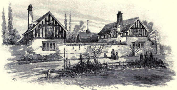
The Stables, Hare Hall, Romford, Essex, W. H. SETH-SMITH, F.R.I.B.A., Architect.
