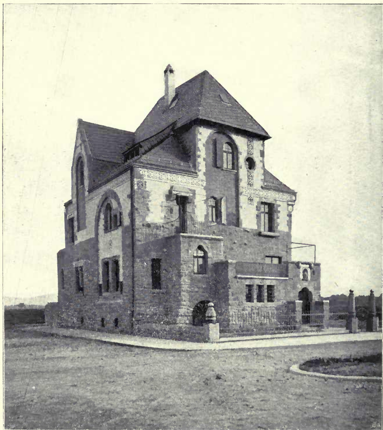
Haus Billing, Eisenlohr Strasse, Karlsruhe, HERMANN BILLING (BILLING AND MALLEPREIN), Architect, Karlsruhe. (For Plans, see p. 123.)
