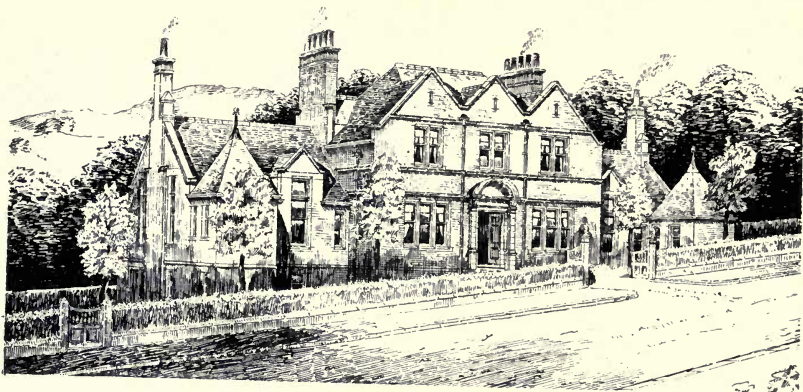
525. Skipton and District Hospital , EDWARD C. H. MAIDMAN, Architect.
