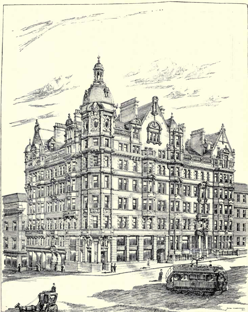
566. Business Premises, Renfield Street and West Regent Street, Glasgow, FRANK BURNET AND BOSTON, Architects.
