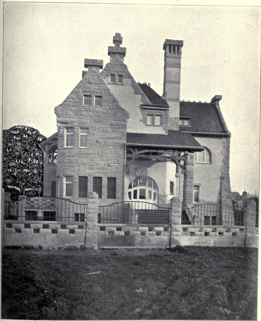
Villa Gerhard Hauptmann, Blasewitz, SCHILLING AND GRAEBNER, Architects, Dresden. (For Plans, see p. 152.)
