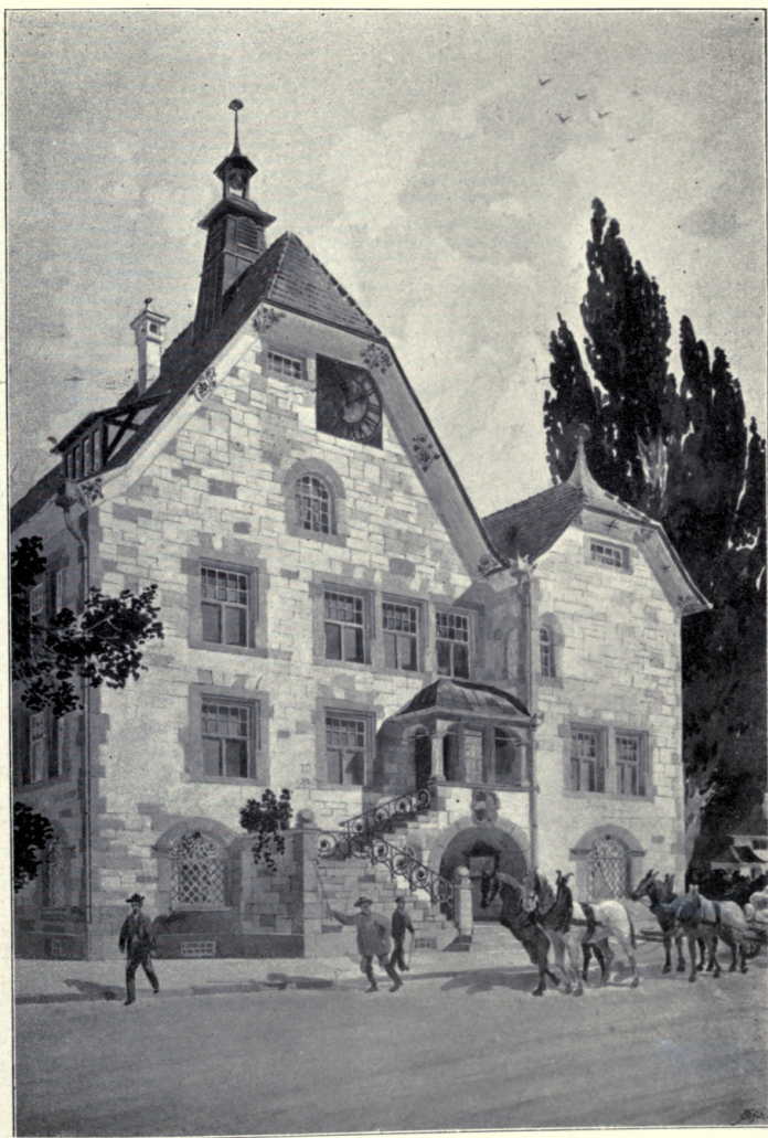
Gemeindefhaus Menziken (Schweiz) , PROFESSOR ROB. RITTMAYER, Architect, Winterthur. (For Plans, see p. 134.)
