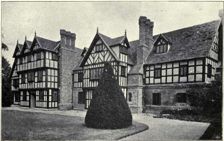
Severn End, Worcestershire, as Restored, LEWIS SHEPPARD AND SON, Architects. (For Plans, see p. 50.)
