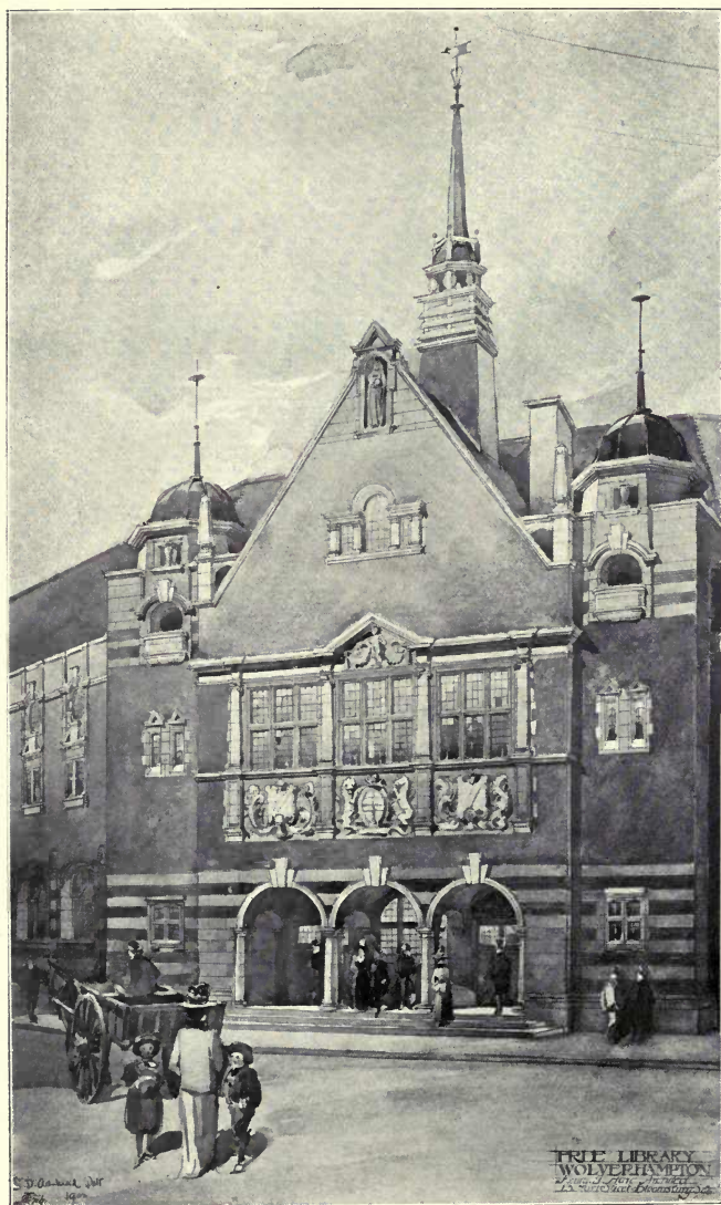
1810. Free Library, Wolverhampton , HENRY T. HARE, F.R.I.B.A., Architect. (For Plans, see p. 33.)
