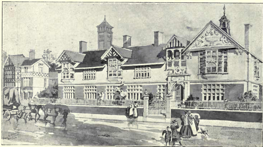
1729. Altrincham Council Offices, HENRY GOLDSMITH, Architect. (For Plan, see p. 104.)
