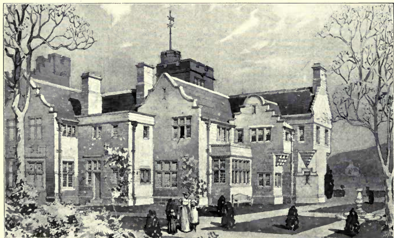
Dalston Hall, Cumberland , JOHN W. BENWELL, A.R.I.B.A., Architect. (For Plans, see p. 141.)
