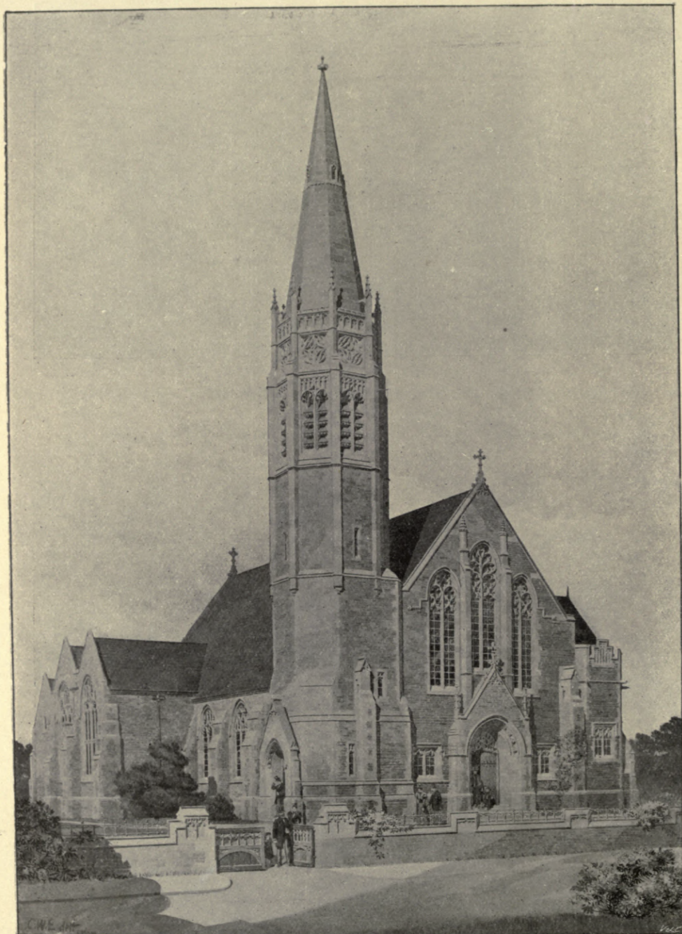
1895. Wesleyan Chapel, Crosby, near Liverpool , J. FRANCIS DOYLE, Architect. (For Plan, see p. 31.)
