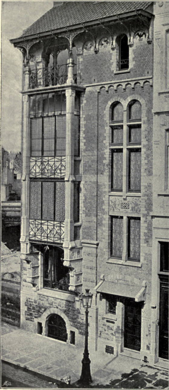
Rue de Facqz, 63, Brussels, P. HANKAR, Architect, Brussels.
