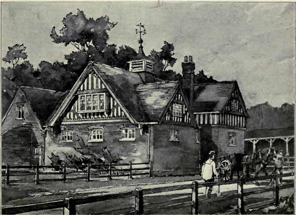
1704. Stables, Matfield, Kent , EDGAR S. UNDERWOOD, Architect.
