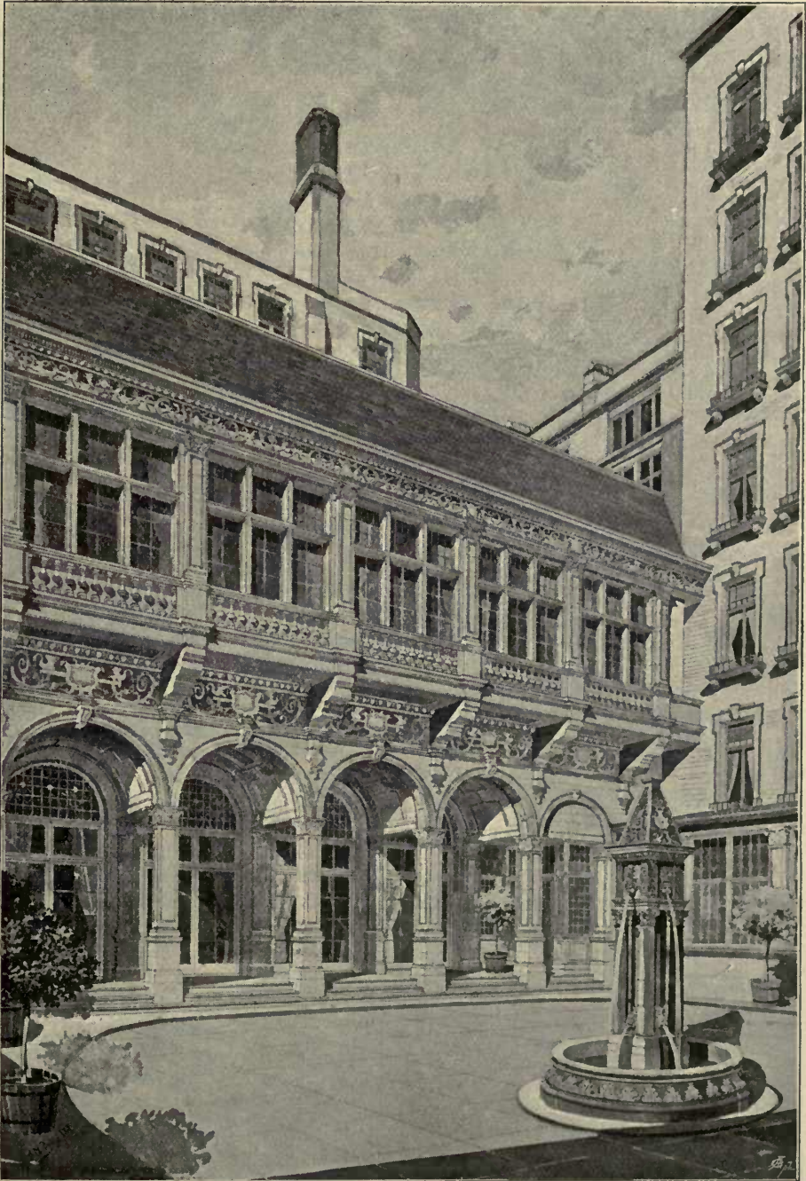
1850. Additions to the Savoy Hotel , T. E. COLLCUTT, F.R.I.B.A., Architect.
