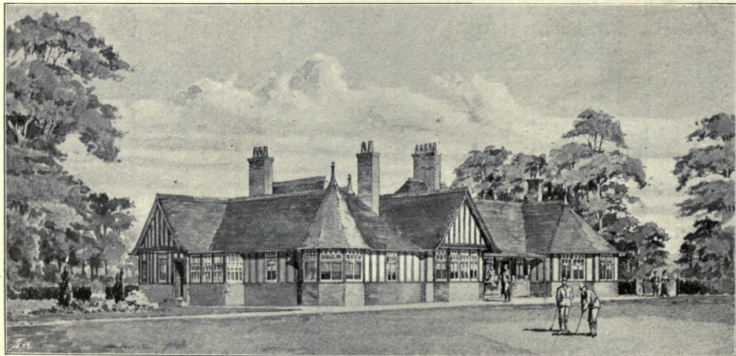
588. Duddingston Golf Club House, Extension for the Insurance and Banking Golf Club , COOPER AND TAYLOR, Architects. (For Plan, see p. 55.)
