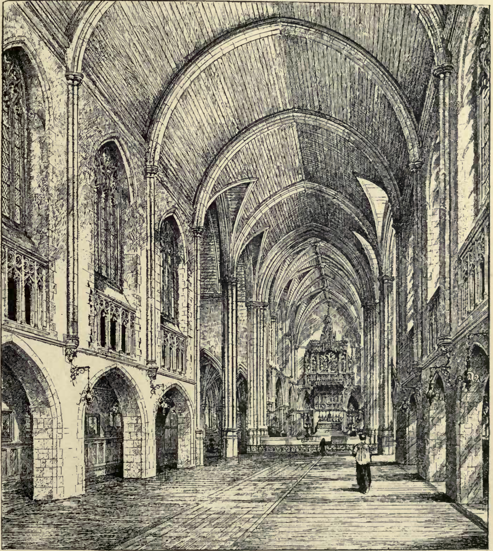
1803. St. Alban's Church, Blackburn, EDWARD GOLDIE, Architect.
