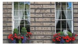
Doors, Windows, Hardware & Shutters
