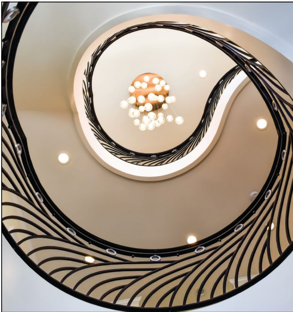
This custom designed, hand forged wrought iron staircase railing by Heritage Metalworks is intricately assembled, featuring Gothic arches and finished with a hammered texture. (Photo by Don Pearse Photography, Inc.)
