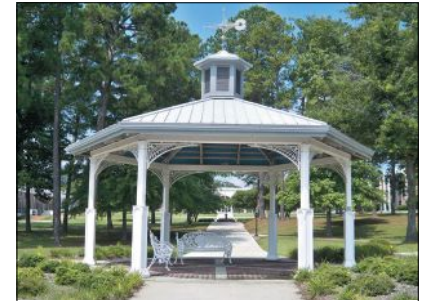
Robinson Iron designed and installed this custom gazebo of cast iron and fabricated water-jet-cut steel for the Central Alabama Community College in Alexander, City, AL.
