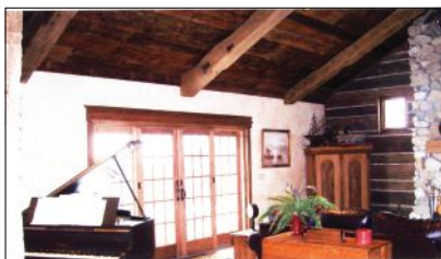
Antique roofer boards, hand-hewn beams, chinked barnwood and recycled window and door trim from Carlson's Barnwood were used to create this charming room.
