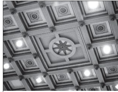
NIKO fabricated and installed these pressed-metal coffers.
