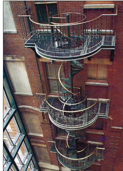
Stairways designed and manufactured this 55-ft.-tall spiral metal staircase with a bronze handrail.
