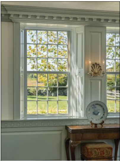
Traditional 18th-century 6" x 8" repurposed crown glass with built in raised panel shutters is from Cooper Historical Windows .
