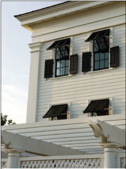
A combination of Chadsworth's Bahama and louvered shutters were used on this structure.
