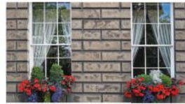
Doors, Windows, Hardware & Shutters
