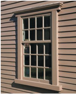
Architectural Components restored the windows for the Jacob Whittemore House at the Minuteman National Historic Park in Lexington, MA.
