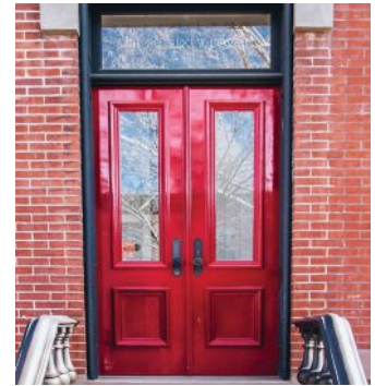
These vibrant red glazed and paneled doors were commissioned to replace a single door with a double-leaved entry doors on a 1880's Park Slope brick row-house by Brownstone Doors .
