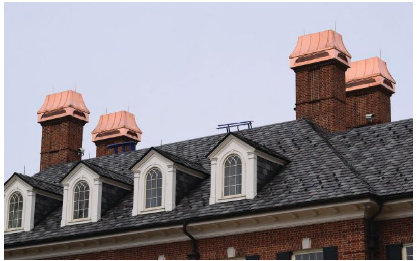
NIKO Contracting created the chimney caps for this home.
