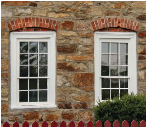
Glass interior storm windows from Innerglass Window Systems solved the draft problems for these windows.
