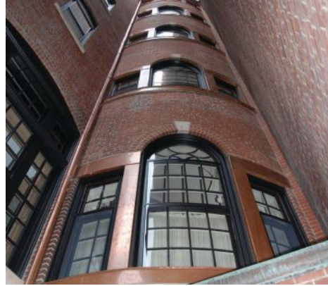
Allied Window supplied the "invisible" storm windows for building in Boston, MA.
