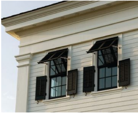
A combination of Chadsworth's Bahama and louvered shutters were used on this structure.
