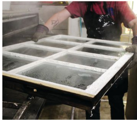
Bagala Window Works uses a steam table to aid in the restoration of windows.
