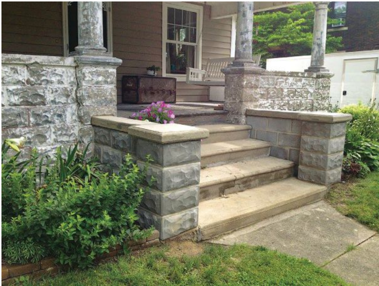
Classic Rock Face Block provided the concrete rock face block to repair these steps.
