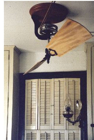
This belt-driven ceiling fan with solid-mahogany blades was supplied by Woolen Mill .
