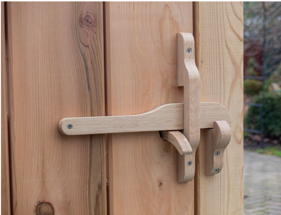
ABOVE A modern reproduction of a traditional thumb latch, showing the interior mechanism.
