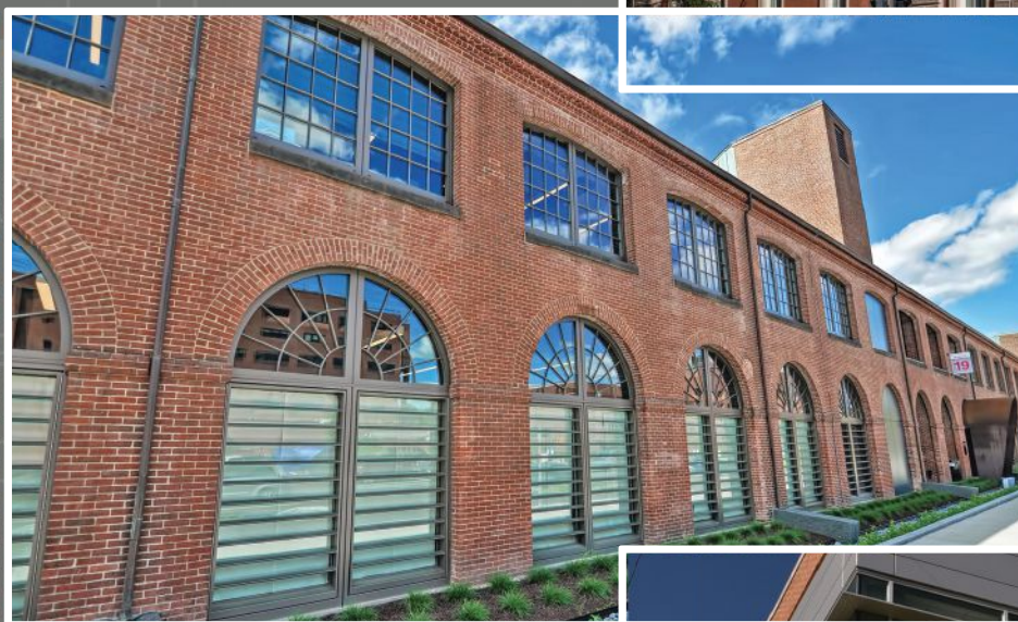
Historic replica windows Springfield Technical Community College: Student Learning Commons
