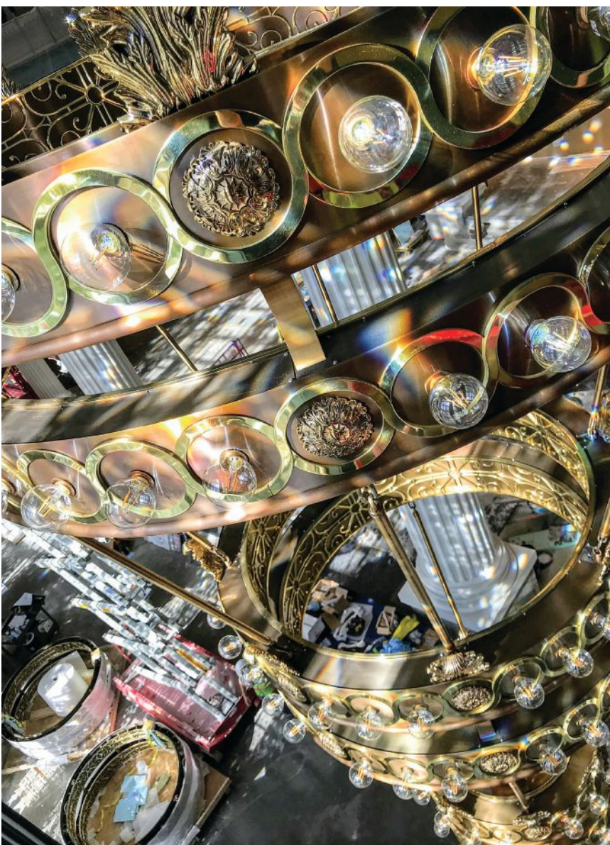
ABOVE A bird's eye view of the assembled and installed chandelier shows not only how the polished brass details meld seamlessly with the patinated rings for a two-tone effect, but also the placement of the ornamental rosettes. All components are designed to reflect illumination down to floor level in a shifting shower of light as viewers pass underneath.
