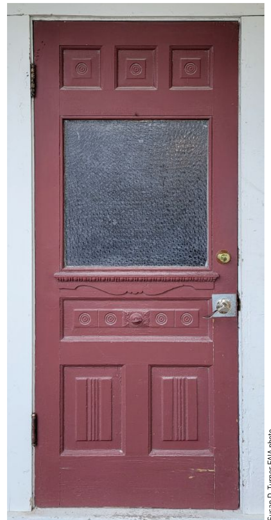
RIGHT An original entry door completely intact, aside from the jarring new hardware which spoils the appearance.
