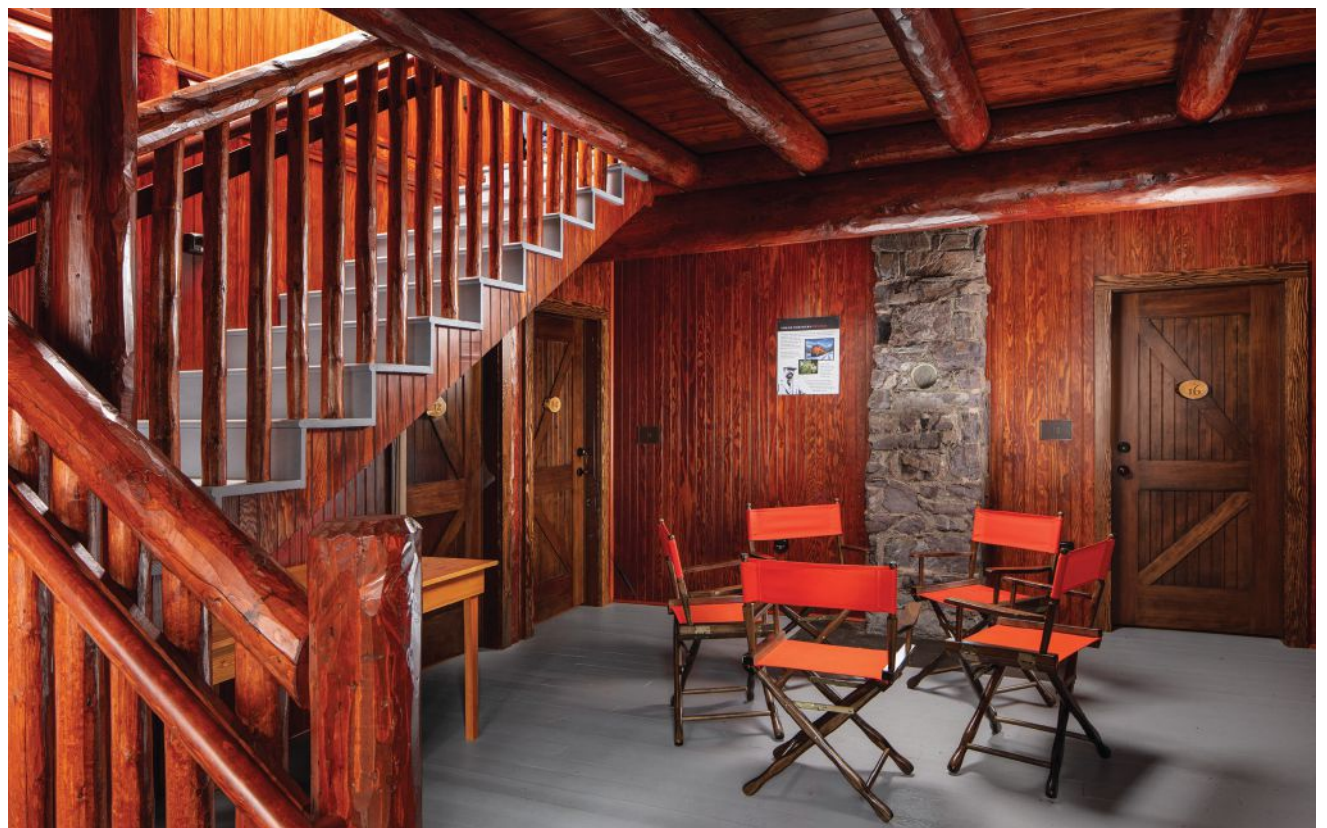
ABOVE The staircase in the chalet's lobby was reconfigured to meet current code.
