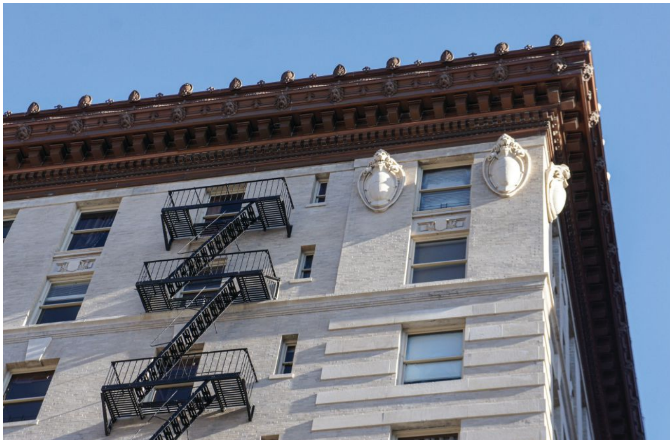
LEFT The Hadrian, shown from the front, with the new cornice.
