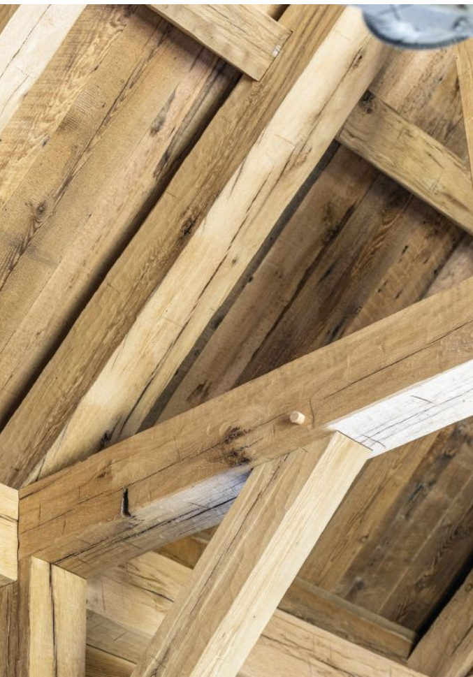
ABOVE Maine Post and Bean did the timber framing.
