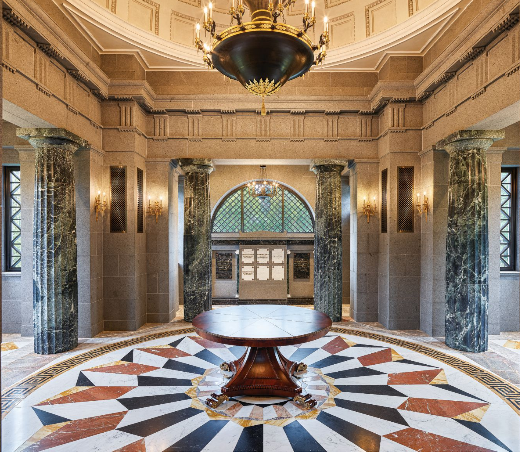
ABOVE The floor pattern, based upon a design in Schinkel's Glienicke Casino in Potsdam, and crafted by Kenneth Castellucci & Associates Inc., features 7 species of Italian and Spanish marbles. The Verdi Alpi columns in the interior were a nod to Daum's employer after graduate school, American Classicist John Blatteau, a founder of Classical America who had placed green Doric columns in a Board Room for Rigg's Bank in Washington, DC.
