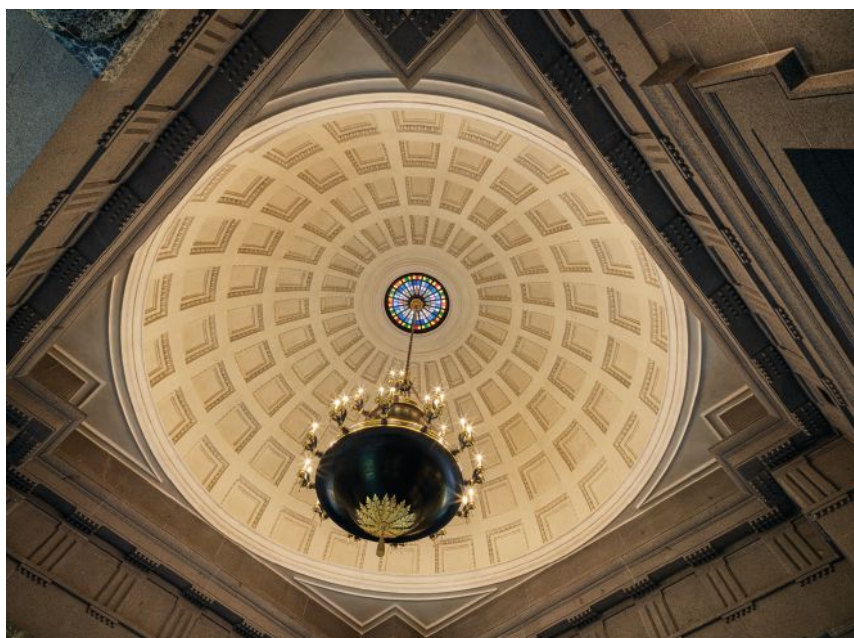
ABOVE Daum's design included the coffered dome symbolizing the 24 hours of the day, fabricated by Foster Reeve & Associates, and the laylight, fabricated by Wiemann Metalcraft depicting a setting sun in an evening sky.
