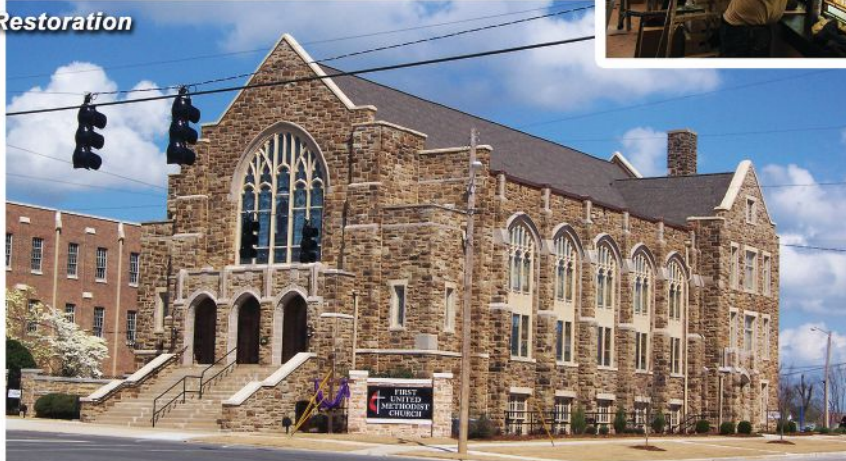
Before and after photos of the F4 tornado damage to the First United Methodist Church of Cullman, Alabama restored by Bovard Studio Inc
