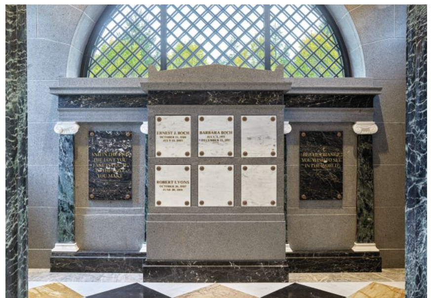
ABOVE The Columbarium fabricated in Cold Spring Charcoal Granite with Portoro Black and Gold base, frieze and plaques, and Verdi Alpi Ionic pilasters with Bianco Carrara capitals and bases, has space for six urns. The form recalls funerary stelae from Greek Antiquity. The inscriptions were selected by the owner.
