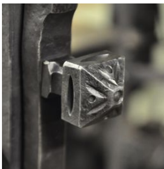
ABOVE Decorated knob of the manually operated and lockable cremone system.
