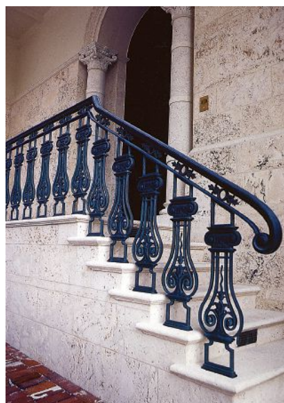
Historical Arts & Casting, Inc. fabricated this traditionally styled, cast-bronze railing.
