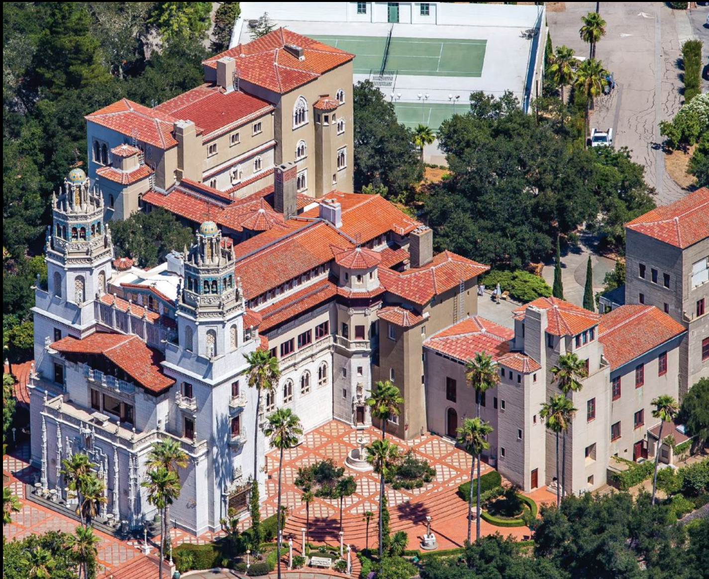
Hearst Castle: Casa Grande, San Simeon, CA - 21st Century Major Renovation
