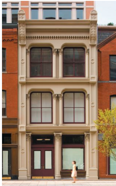
Robinson Iron cast and fabricated this new storefront façade in aluminum to match the surrounding historic neighborhood in Washington, DC. Click on No. 3240
