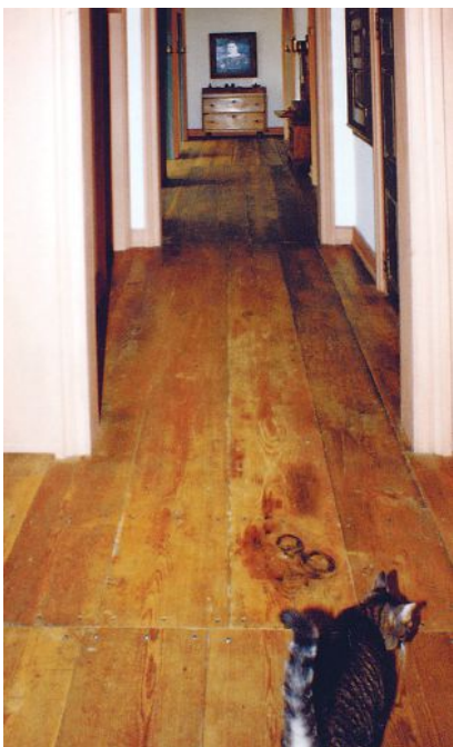
Resawn flooring from Sylvan Brandt is cut from old beams to match the grain and character of antique floors. Click on No. 3950
