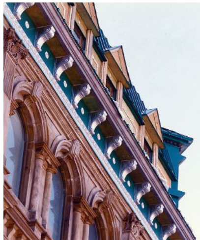
This stamped sheet-metal cornice was fabricated by W.F. Norman . Click on No. 520
