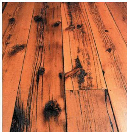
Conklin's Authentic Antique Barnwood supplied this skimmed pine and hemlock flooring, which is made from reclaimed wood.
