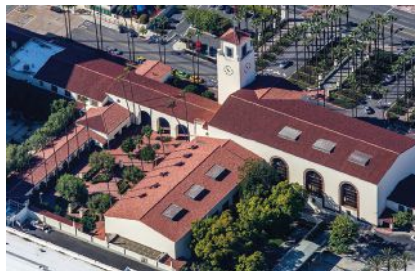
MCA Clay Roof Tile was selected for the renovation of the historic LA Union Station, preserving the original design by creating tiles based on the original historical tiles. Built in 1939, LA Union Station is widely regarded as "the last of the great train stations," its architecture and design an iconic presence in the Los Angeles landscape. Click on No. 2101
