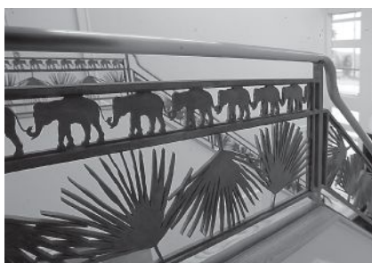
This elephant motif railing was created by Robinson Iron using water-jet-cutting technology. Click on No. 3240
