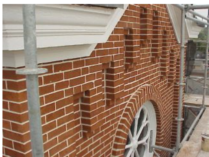
LimeWorks.us provides restoration and repointing services for masonry projects.
