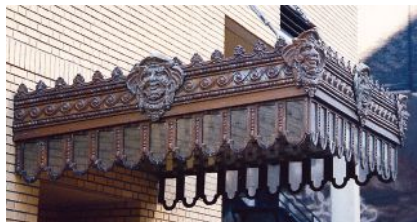
This decorated sheet-metal canopy was fabricated by W.F. Norman . Click on No. 520
