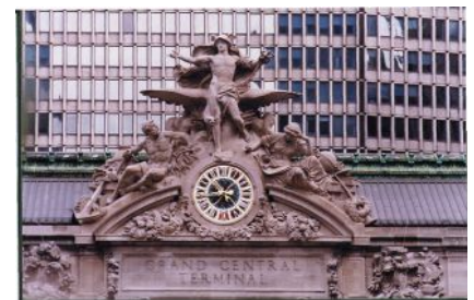
Rohlf's removed and restored the Tiffany clock at Grand Central Terminal, NYC, replicating missing parts. Click on No. 6240
