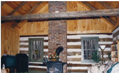
This 45x34-ft. barn was constructed by Sylvan Brandt using four bents and eight major outside posts, most of which are hand-hewn hardwood. Click on No. 3950
