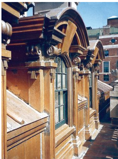
NIKO Contracting restored these copper dormer surrounds. Click on No. 8300
