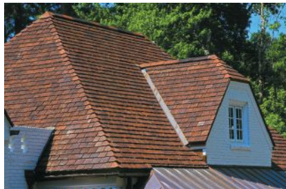
Ludowici's black-mist Colonial Tile and bonnet hip plates were used on this roof. Click on No. 2760
