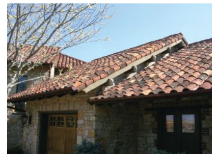
Tile Roofs supplied 8,500 sq.ft. of salvaged weathered Mission tile for this new home.
