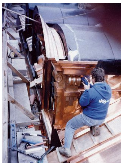
The replication of exterior ornamental copwork is a specialty of NIKO Contracting Co. Click on No. 8300
