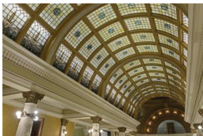
Conrad Schmitt Studios removed, conserved, re-leaded and reinstalled the stained-glass of the South Dakota State Capitol; the glass in this barrel-vaulted ceiling and the glass in the rotunda dome went through an extensive conservation process. Click on No. 8040
