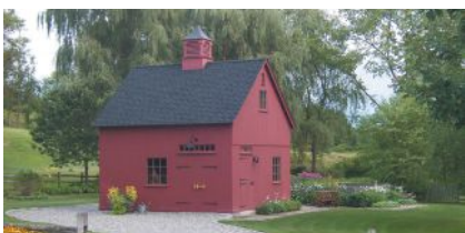
This 18x20-ft. post-and-beam barn was built with a kit from Country Carpenters using stamped and graded timbers and premium-grade, kiln-dried siding.
