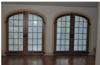
These elliptical arched-top French doors with double pane insulated glass were fabricated by Illingworth Millwork . Click on No. 1690
