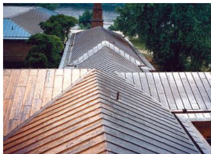
NIKO Contracting Co., Inc. installed this batten-seam and flat-lock copper roof. Click on No. 8300
