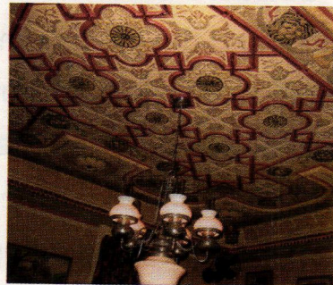
This Oriental-style ceiling was created using pressed-tin panels from W.F. Norman Corp.
