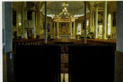
These cast-iron radiators were restored by Ecorad .
