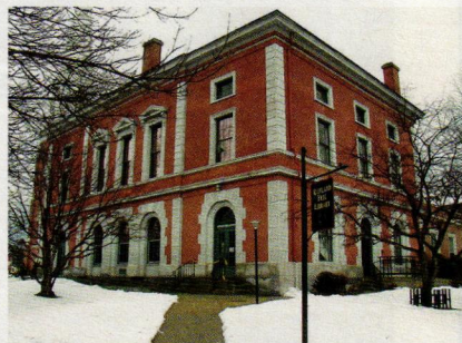
Innerglass Window Systems supplied interior glass storm windows for this historic building.
