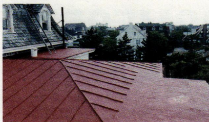
This metal roof has been treated with a water-proofing, elastomeric Acrymax coating from Preservation Products.
