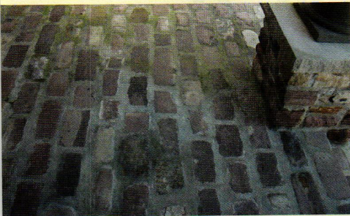
Avian Historical Bricks supplied the reclaimed Old English cobblestones with rounded tops for this walkway.
