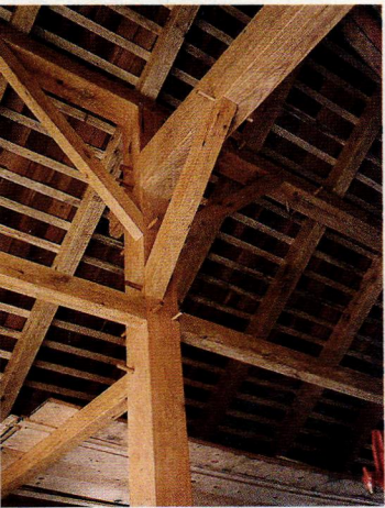
Architectural Timberworks designs, joins and fabricates timber-frame structures, using traditional post-and-tenon joinery.
