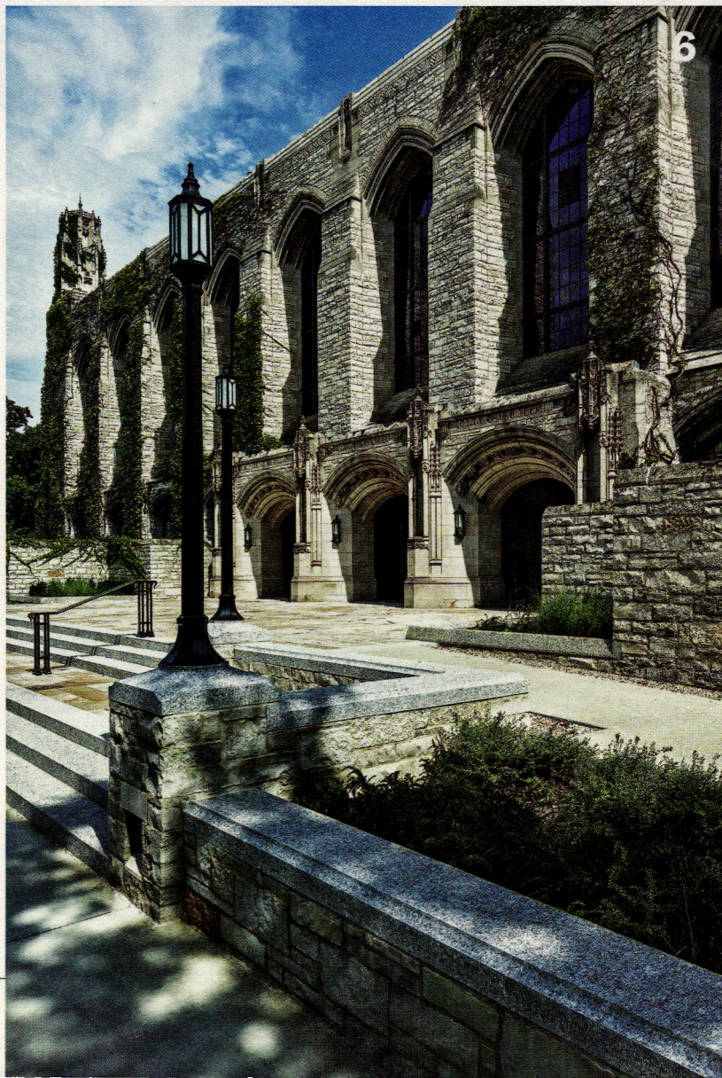
6: The landscaping of the new entry plaza included retaining walls of Wisconsin Lannon stone capped with granite, and a pair of sloping ramps behind them for ADA access.
