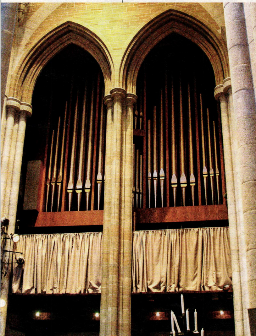
A before view of the twin main arches shows the decommissioned freestanding organ pipes and how the new woodwork will have to integrate with the clustered stone piers. All photos: Len Levasseur
