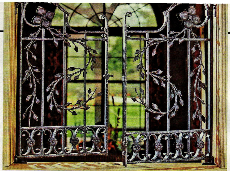
The Minnesota Governor's residence was designed by architect William Channing Whitney and built 1910-1912 for Horace Hills Irvine, a lumberman and lawyer in St. Paul, MN. The original home had two interior window openings filled with ironwork. At some point, the metalwork disappeared. The new forged steel gates were replicated by Robert Walsh and his colleague Tom Latane, based on a 1920s photo taken in the residence.
