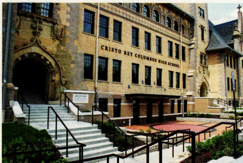
CLOCKWISE FROM TOP LEFT: A view of the east elevation. The building now has historically appropriate new windows and a new roof.
