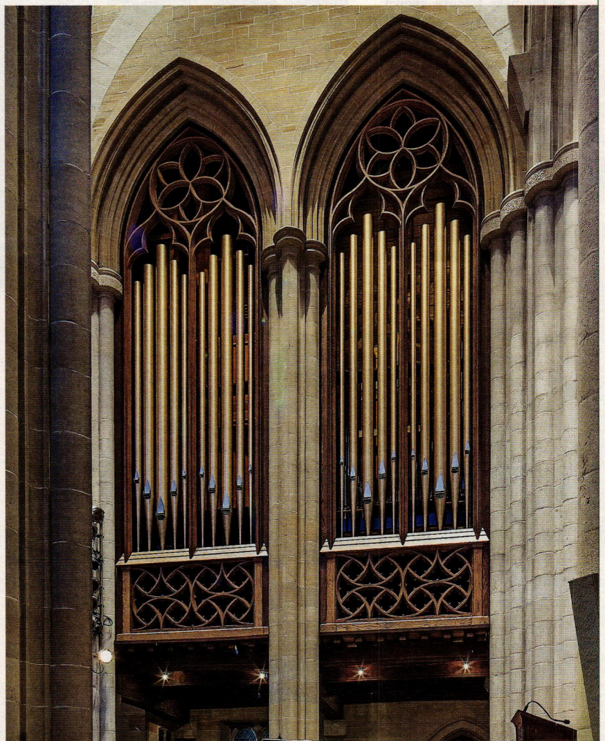
The completed main arch facades. As seen by the congregation, the white oak woodwork harmonizes with the Gothic cathedral architecture without upstaging stonework or obscuring the new pipe organ.
