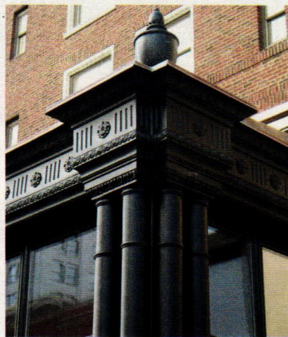
Wagner Foundry cast this aluminum storefront for The Pentland Hotel in Grand Rapids, MI.
