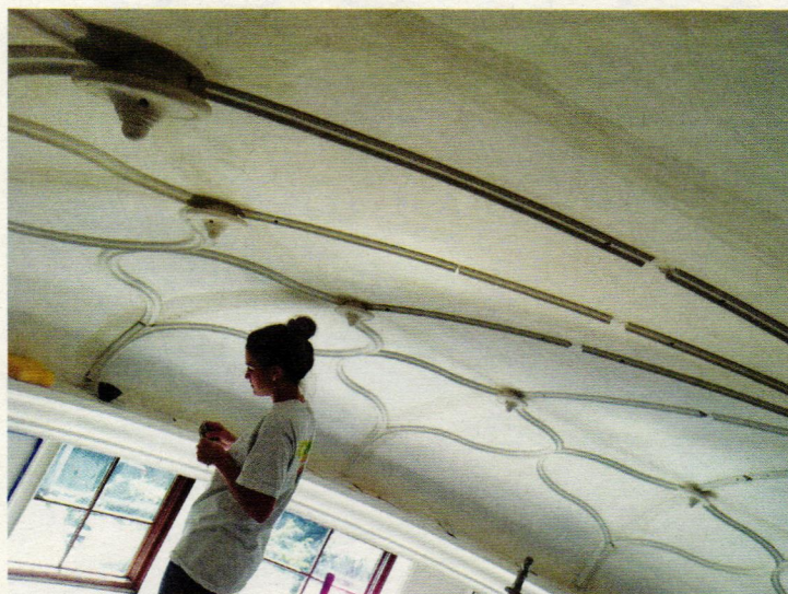
A student apprentice learning to affix and join plaster tracery elements on a plaster dome
