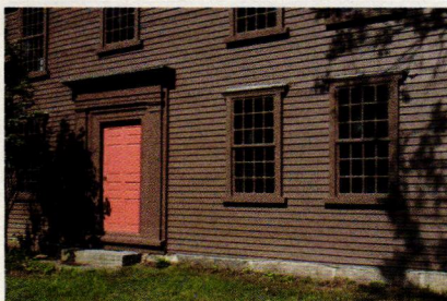
Architectural Components restored the windows, doors and reproduction 18th-century hardware for the Jacob Whittemore House at the Minuteman National Historic Park in Lexington, MA.
