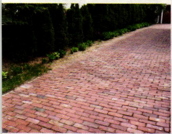
Historical Bricks supplied its reclaimed English Cobblestones for this driveway in San Francisco, CA.
