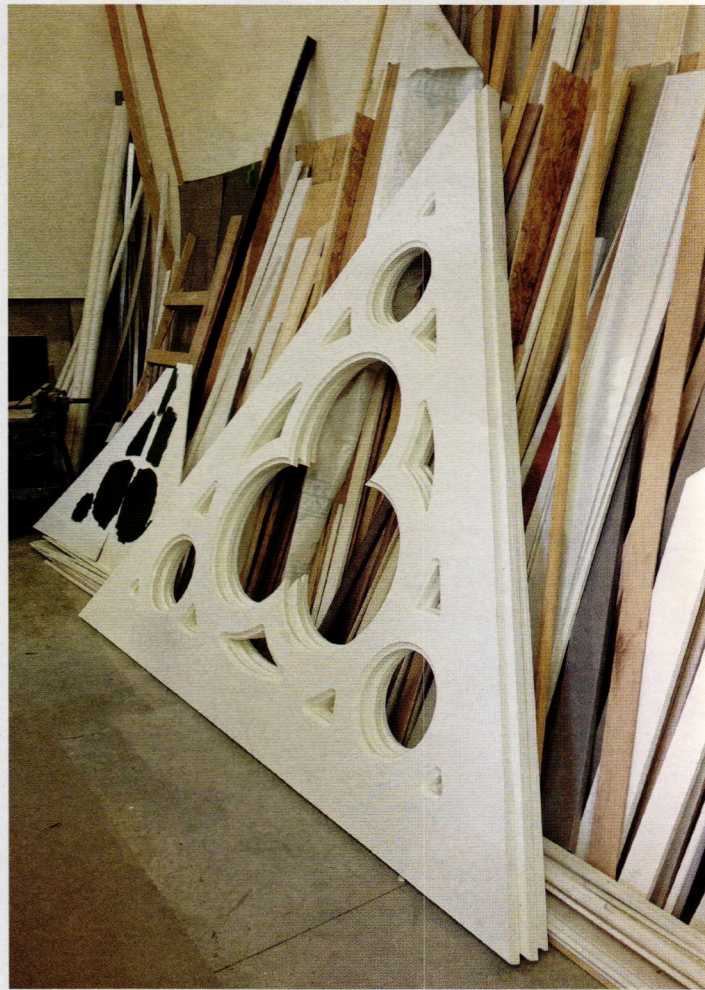
ABOVE: The rotting wood on the tower was removed, and taken to Nugent Builders' shop in Rockford, MI, where it was measured, photographed and reproduced. Each side of the tower measure 10 ft. wide and the trefoils are 6 ft. wide.
