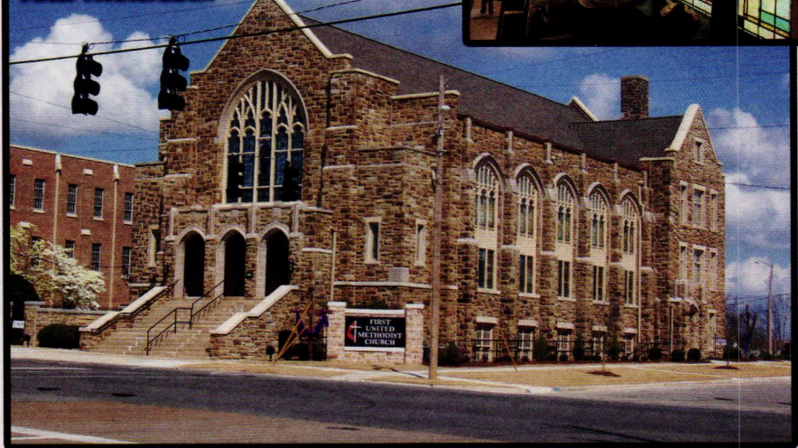
Before and after photos of the F4 tornado damage to the First United Methodist Church of Cullman, Alabama restored by Bovard Studio Inc
