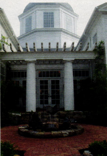
Chadsworth's fluted Greek Doric fiberglass columns, measuring 24 in. by 125 in., are used in the entryway of the Poland Branch Library in Sand, OH.
