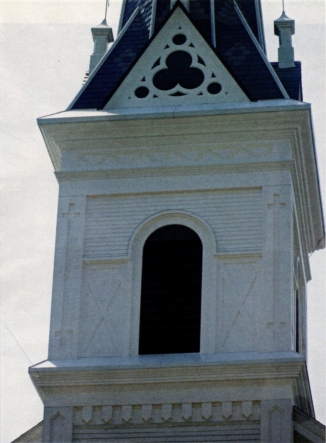
ABOVE: The rotting wood on the tower was removed, and taken to Nugent Builders' shop in Rockford, MI, where it was measured, photographed and reproduced. Each side of the tower measure 10 ft. wide and the trefoils are 6 ft. wide.
