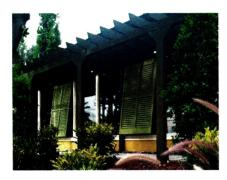
Chadsworth's custom exterior Bahama-style shutters, made from pultruded fiberglass, are installed on an Olive Garden restaurant in Orlando, FL.
