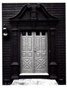
This reproduction broken-pediment doorway with cross-buck doors and bulls-eye glass was fabricated by Architectural Components.
