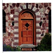
Heart Wood Fine Windows & Doors fabricated this 2 ¼-in. thick mortise-and-tenon solid-wood door out of sawn white oak to replicate the original door made 100 years ago.
