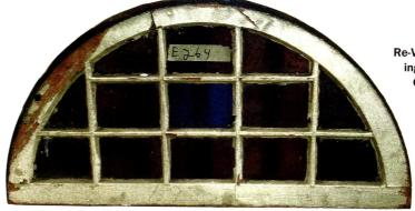
Re-View restored 340 wood windows, including 126 curved units, for the Knox County Courthouse in Knoxville, TN. The windows are wood with aluminum storms on the exterior. In some cases where the original windows had been replaced in the past, the replicas were built to match the originals. Photos: courtesy of Re-View
