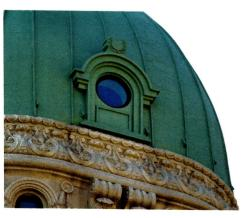
Gotham Metalworks fabricated this precision plasma-cut replication domed roof for a NYC landmarked building.
