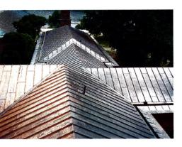
NIKO Contracting Co., Inc. installed this battenseam and flat-lock copper roof.
