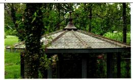
This gazebo features W.F. Norman Corp's style A shingles with its continuous hip finish and a custom-made finial on top.
