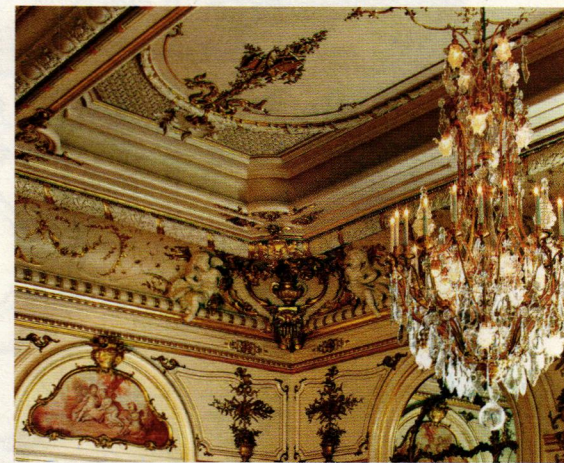
John Canning Studios restored and conserved the ornamental plaster and elaborate murals throughout the Cosmos Club Warne Ballroom in Washington, DC.
