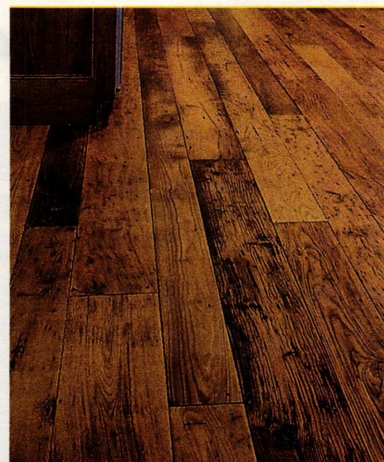
This random-width chestnut flooring was fabricated from hand-selected, re-milled lumber from Chestnut Specialists.
