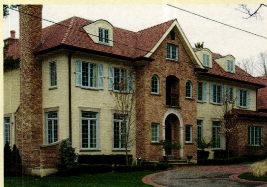
This new home in Glencoe, IL, features 8,000 sq. ft. of new fire-flashed shingle tiles supplied by Tile Roofs .
