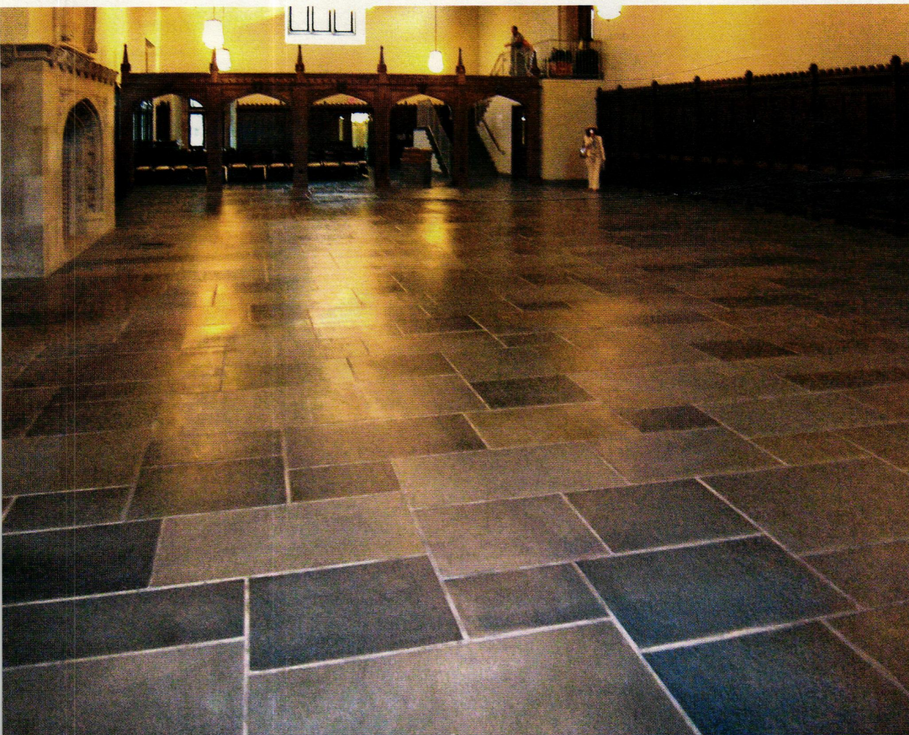
Bluestone flooring from Endless Mountain Stone was specified for this building at Princeton University.
