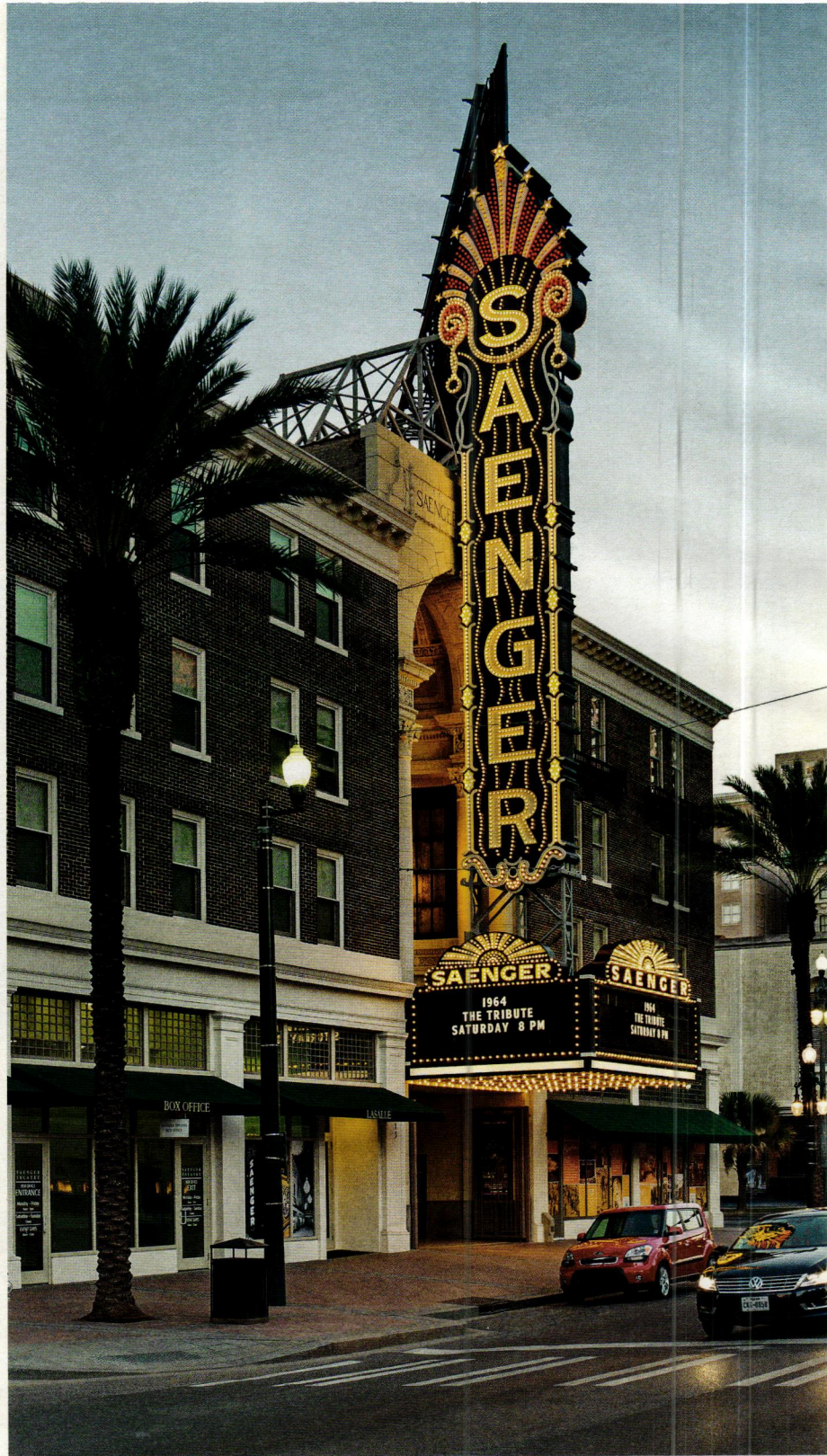
RIGHT: The front Saenger sign, copied from photos of the original, makes a show-stopping and car-stopping statement on Canal Street.
