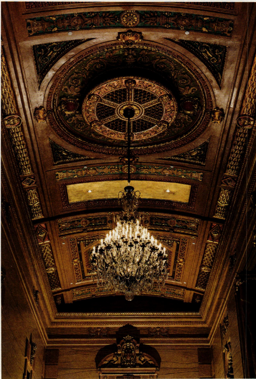
ABOVE: The ornate architectural detailing was restored to its original splendor.
