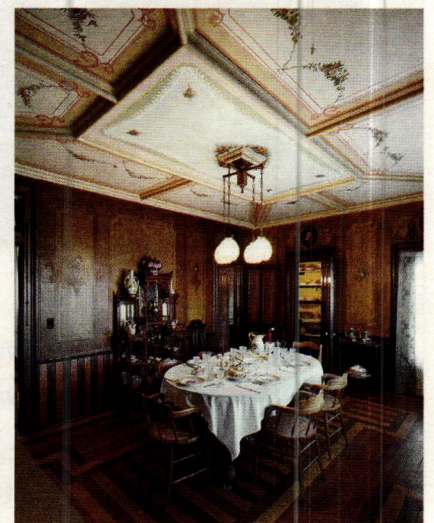
EverGreene Architectural Arts restored the decorative painting in the ceiling at the 1865 Tinker Swiss Cottage in Rockford, IL.
