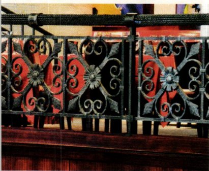
Wiemann Metalcraft designed this aluminum and forged steel railing system for the Packard Building in Philadelphia, PA, to be sympathetic to the historic Yellin work found elsewhere in the building.
