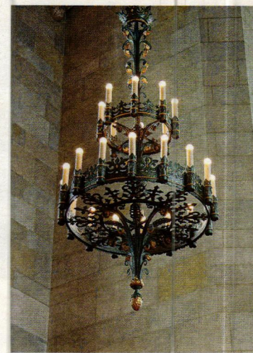
Crenshaw Lighting restored the 42-in. dia. x 9-ft. tall, two-tier, cast-bronze fixtures in the William W. Cook Research Library at the University of Michigan.
