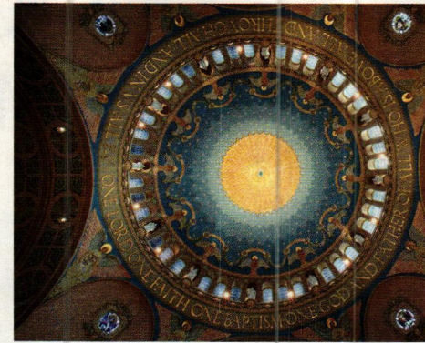
Conrad Schmitt Studios restored the decorative painting for St. James Catholic Church in Louisville, KY, including the faux mosaic on the ceiling.
