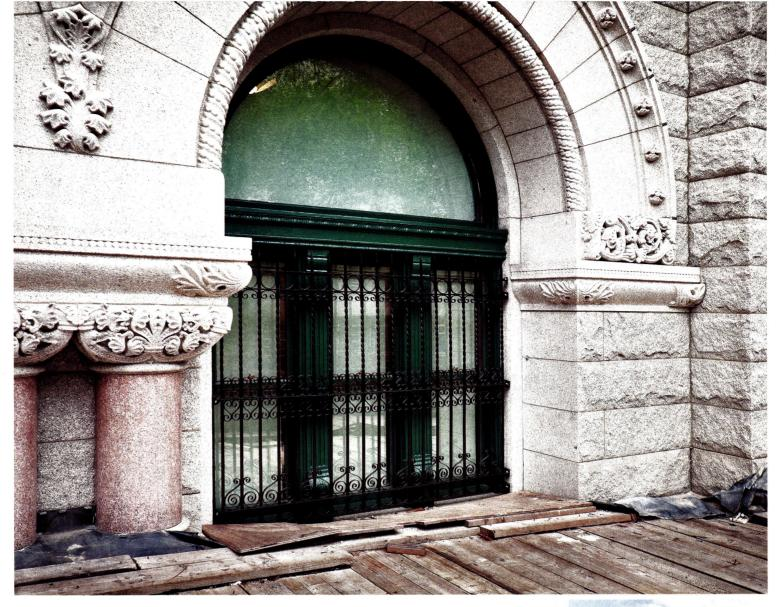
ABOVE: A typical window restoration in the granite building involved restoration of the wood frame in place. The wood sash was restored and retrofitted with insulated glazing and the upper sash was fixed in place. All sash weights and hardware were restored and new weatherstripping was added.
