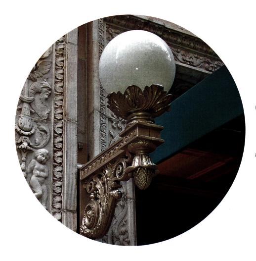
Ball and Ball repaired and refinished this original fixture on a New York City apartment building. After rewiring it, the company installed LED lamping in the owner-sourced glass globes. Photo: Bill Ball
