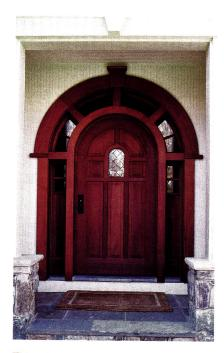
This raised-panel door was custom fabricated by **Kolbe & Kolbe Millwork** in mahogany.
