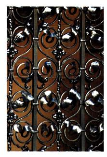
The Renaissance forgework reproduction for the Dakota inner courtyard gate in New York City was created by **Fine Architectural Metalsmiths**; it includes repoussed center rosettes and strongly arched infill leaves, collared joinery and scrolls, which end in a one, two or three leaf pattern.
