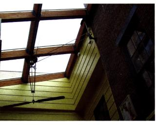
Woolen Mill Fan Co. manufactured the Moa, a belt-andpulley fan system with an optional line shaft, for Fisher's Restaurant in York, PA. Click on no. 316.
