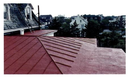
This metal roof has been treated with a waterproofing, elastomeric Acrymax coating from **Preservation Products**. Click on no. 8180.
