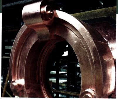
**Gotham Metalworks** created this copper-covered oriel window, taking into account the complex angular geometry and the integrity of the building's original architecture. Click on no. 2042.
