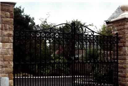
CLOCKWISE FROM LEFT: This iron gate for a 12-ft. opening was cast in one piece by Wiemann Metalcraft; it was installed on in-ground hydraulic operators. Photo: courtesy of Wiemann Metalcraft
