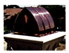
EJMcopper Inc. fabricated this chimney cap, which includes a bug screen.
