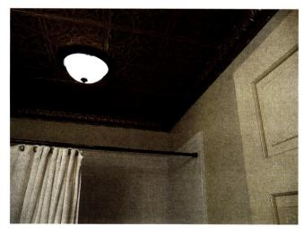
This hand-painted faux-finish metal ceiling was fabricated and installed by Metal Ceiling Express.
