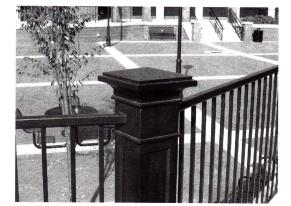
This custom cast-iron stanchion was fabricated by O.K. Foundry.
