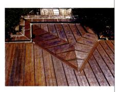
NIKO installed this batten-seam and flat-lock copper roof for an historic building.
