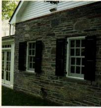
These raised-panel shutters from Shuttercraft with propeller holdbacks were installed on a stone-sided home with recessed windows.
