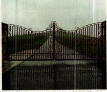
These estate gates featuring scrollwork and ornate designs were fabricated by Lodi from architectural-grade aluminum; the overall span of the 13-ft.-tall gates is 36 ft.
