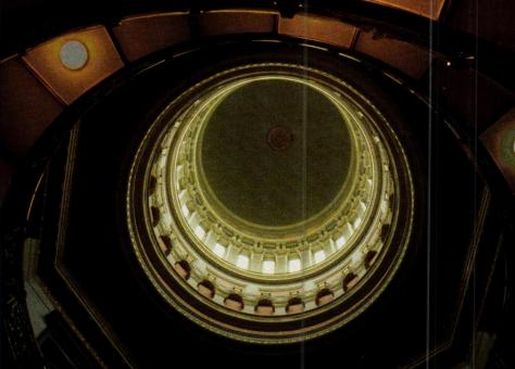
Constructed in 1792, the New Jersey State House gained an 80-ft. high rotunda and dome in 1885, but by the 1990s, the flaking gold leaf was only a symptom of larger deterioration. JHPA prepared construction documents for repairing the cast iron in the rotunda (above) and structural steel in the dome, as well as interior finishes and lighting.
