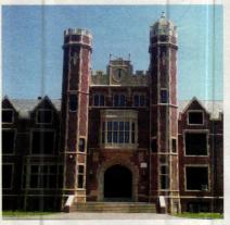
On Staten Island, NY, Graciano Corp. completed extensive historic masonry conservation at Wagner College's Main Hall; it included restoration, waterproofing and exterior cleaning of the 1929 precast-concrete building, as well as rebuilding parapets and copings, reconstructing the top half of two five-story Gothic-style turrets, and replacing the dome that surmounts one of the turrets.
