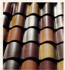
When replacing the terra-cotta roof of the Breakers mansion in Newport, RI, Boston Valley Terra Cotta used 35,000 field tile and approximately 4,000 special-shaped fittings.
