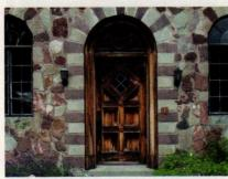
HeartWood Fine Windows & Doors made this 21/4-in. thick mortise-and-tenon solid-wood door of sawn white oak to replicate the original door made 100 years ago.
