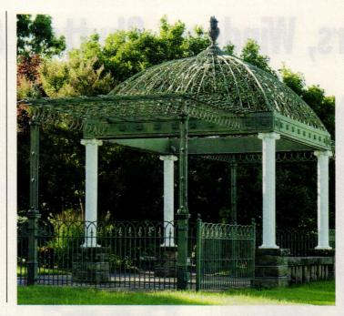
Wiemann Metalcraft fabricated this gazebo, fence and trellis in cast and wrought iron.
