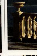
Haddonsone's caststone balustrading can be formed into straight, ramped, curved and spiral configurations and is used on steps, balconies and parapets.
