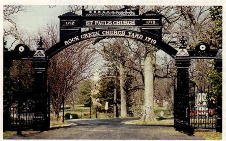
Architectural Iron restored this massive cast- and wrought-iron main gate for the Rock Creek Cemetery in Washington, DC.
