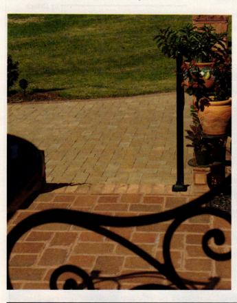
Pine Hall Brick's CityCobble pavers are tumbled after firing, giving them a cobbled look; the pavers exceed ASTM standards for strength and durability and will not fade.
