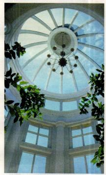
Oak Leaf glass domes feature insulated curved double-glazing with laminated and other performance enhancing glass, curved laminated hardwood internal rafters and ring beams and a proprietary low-maintenance extruded-aluminum classically profiled capping system.
