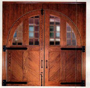
The renovation of this historic fire house included eco-friendly strap hinges and back plates (37% recycled steel in content and coated with a no VOC powder coat) from Richards-Wilcox.
