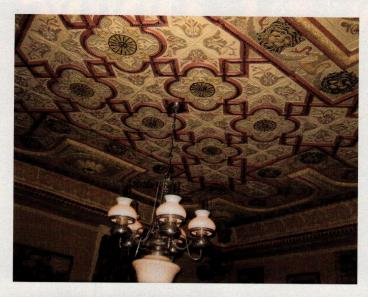
This Orientalstyle ceiling was created using pressed-tin panel from **W.F. Norman**.
