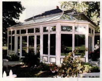
Glass House fabricated and installed this mahogany-frame octagon-ended conservatory with leaded glass, dentil molding, french door sets and casement windows, raised panel base wall, decorative ridge cresting and finials, and stateof-the-art glazing.
