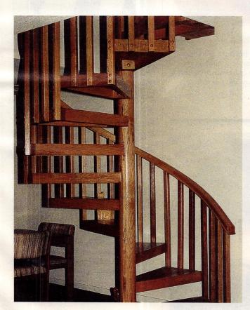
Goddard fabricates both wood and metal spiral staircases.
