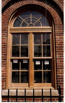
This double-hung window unit with a fixed-arch fan was constructed by Artistic Doors & Windows with mortise-andtenon joinery.
