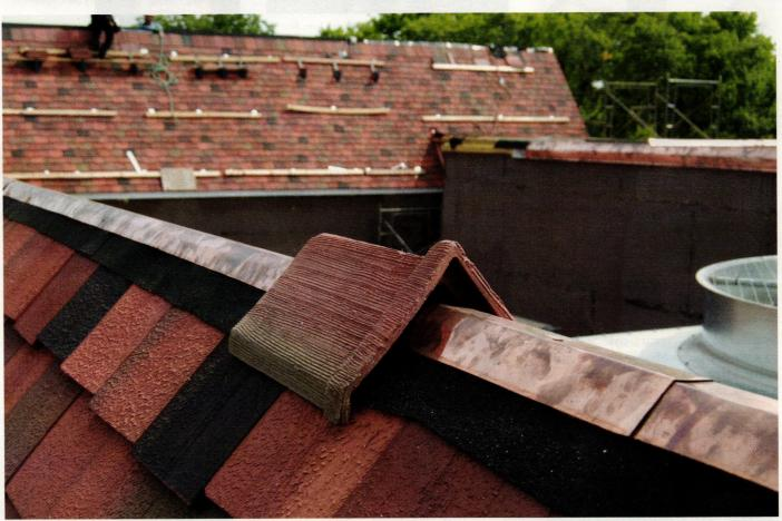
Roofing accessories, such as ridge tile, were also replicated. The original ridge tile features a very thick collar and heavy scoring, both of which Ludowici was able to match.
