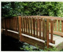
This prefabricated pedestrian bridge is one of many styles available from Western Wood Structures; it is made from second-growth, glue-laminated wood, a primary building material made from a renewable resource.
