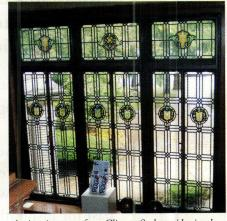
An interior storm from Climate Seal provides insulation while protecting the appearance of this historic window.
