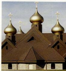
Five onion-style golden domes were custom manufactured and installed by Architectural Fiberglass, Inc. on the Holy Trinity Church in Parma, OH; one measures 18x32 ft. and the other four are 15x26 ft.
