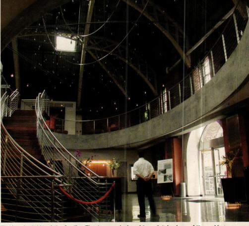
The interior lobby of the Gerding Theater was designed to maintain views of the arching bowstring lattice trusses that span a 100x200-ft clear space.
