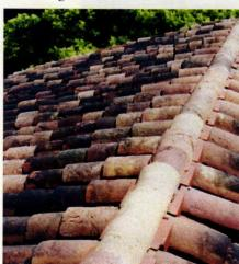
Salvaged clay tile supplied by Tile Roofs was used to create an instant patina on this roof.
