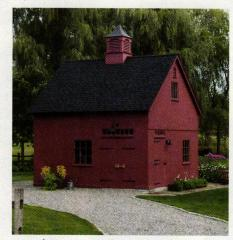
This 1<sup>1</sup>/<sub>2</sub>-story post-and-beam 18x20-ft. barn was built with a kit from Country Carpenters using stamped and graded timbers and premium-grade, kilndried siding.
