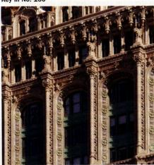
Boston Valley Terra Cotta repaired and restored the terra-cotta facade at 90 West St. in New York City after it was damaged during 9/11.
