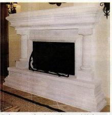
Both custom and stock mantels are available from Aristone Designs in cast stone and GFRC.
