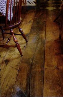
Reclaimed, hand-planed antique chestnut flooring supplied by Old Wood Workshop is available in widths from 9 to 14 in.
