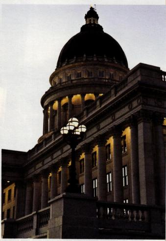
The Utah State Capitol in Salt Lake City recently underwent a seismic upgrade and full exterior and interior restoration by Capitol Restoration Group (CRG). The group's primary goals were to improve life safety through base isolation; efficiency through mechanical upgrades; and to restore and preserve the building's historic finishes and details.
