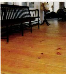
Wide pine flooring from South County Post & Beam is kiln dried, joined straight and ripped parallel.
