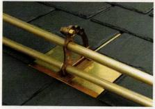
AlpineSnowGuards' model # 502 brass two-pipe snowguard is shown on a synthetic slate roof.
