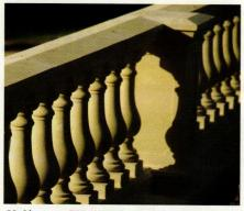
Haddonstone (USA)'s cast-stone balustrading can be formed into straight, ramped, curved and spiral configurations and used on steps, balconies and parapets.
