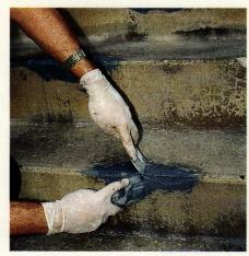
Abatron's Abocrete restoration epoxies can be used to patch various surfaces.
