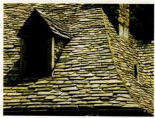
Greenstone Slate manufactures and installs slate roofing in a variety of colors, shapes and sizes.
