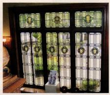
An interior storm from Climate Seal provides insulation while protecting the appearance of this historic window.
