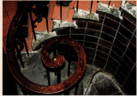
Bright orange quarry tile that had been installed over the bluestone floor was removed so the original stone and tile on the floors and walls could be restored. The stairway that goes to all five floors was also restored.
