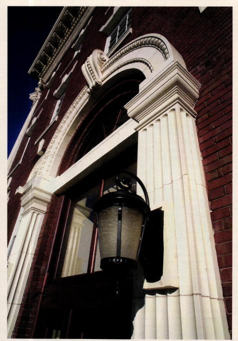
This side entry to the Blodgett Building gives a clear sense of just how meticulous the restoration was: lost terra-cotta ornament was replaced in GFRC, missing bricks were replaced with salvaged vintage brick, and period-style exterior lighting was added. Photo: Mark Thomas Productions
