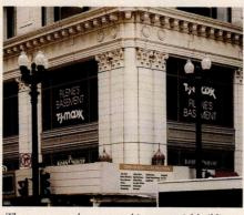
The terra-cotta elements on this commercial building in Chicago were replicated with GFRC elements with technology provided by Ball Consulting.
