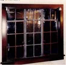
Seekircher, a specialist in steel casement-window adjustment and restoration, rebuilt this window after it was damaged in a storm.
