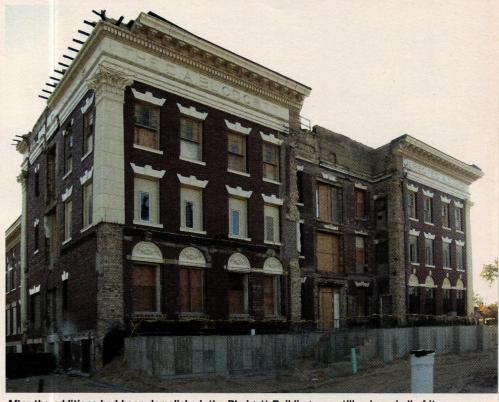
After the additions had been demolished, the Blodgett Building was still only a shell of its former self. "We were making a lot of assumptions about what was going to be there when we removed the newer addition," says Heather DeKorte, project architect, "but once it was removed, for the most part we were actually pleased by how much of it was intact." Photo: Cornerstone Architects
