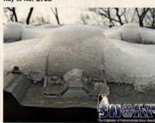
Designed for metal roofs, the Ice Jax II clear polycarbonate snowguard from Snoblox holds 6,388 lbs. of snow when screw mounted.
