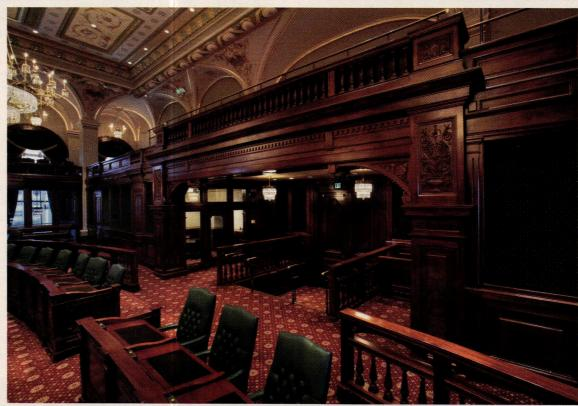
At the back of the House, long-lost brackets have been replicated and carved with foliage, scrollwork and shields.
