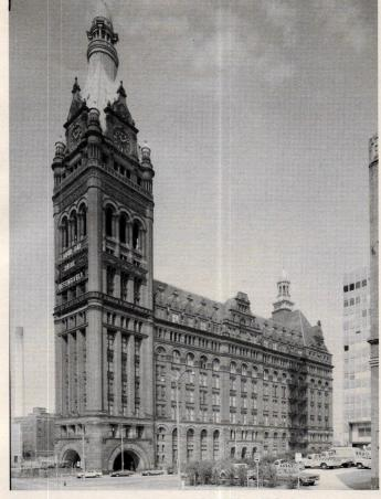
Tower-wrapping signage, shown in this 1970s HABS photo, proved damaging to the masonry and has been removed. But the clock faces, which coal soot had blackened by the 1920s, have been brought back to their original translucence. Photo: Eric Oxendorf, HABS
