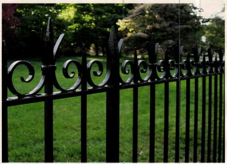
This custom fence was designed and fabricated by Wiemann Ironworks using solidbar steel; to ensure longevity, it was galvanized before urethane coating was applied. Key in no. 1223
