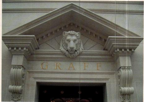
The exterior ornament on this Palm Beach, CA, building was fabricated in French limestone by **Traditional Cut Stone**. Key in no. 2902
