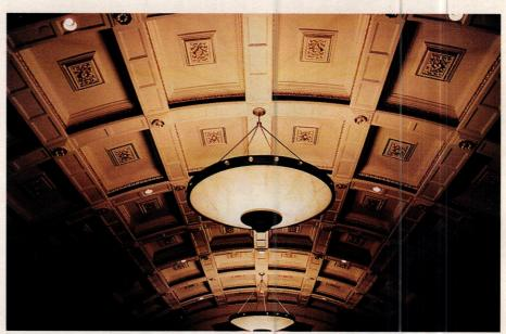
Flex Moulding used polyester resin to create this ornate barrel-vaulted ceiling. Key in no. 4900
