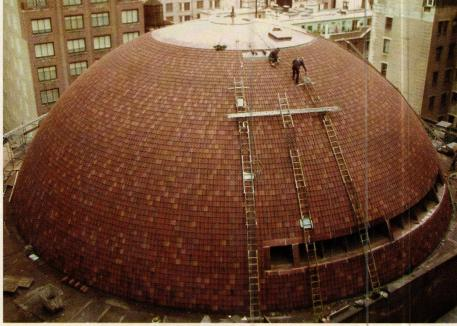
The dome of the New York City Center was originally finished in **Ludowici Roof Tile** in 1923; it was restored with roof tile from the same company in 2004. *Key in no. 2760*
