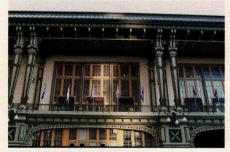
Allen Architectural Metals replicated and restored the cast-iron facade and railings for this 140,000-sq.ft. 1909
