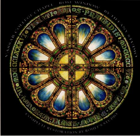
The Tiffany Rose Widow at the Vassar College Chapel in Poughkeepsie, NY, was removed, re-leaded and re-installed by **Rohlf's Stained & Leaded Glass Studio**; the firm also retrofitted the double-glazed steel frame system. *Key in no. 1480*
