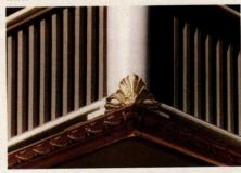
This ornate gutter, fabricated by Classic Gutter Systems, incorporates a hidden adjustable hanger system.
