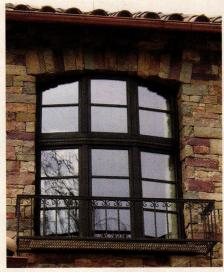
This custom bronze-clad tilt-and-turn window was fabricated by Grabill; it has an antiqued patina and an aged-wood interior.
