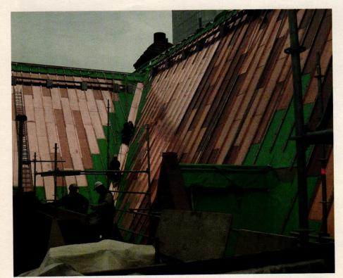
Laying a new copper roof for Old City Hall involved the removal of the old roofing, the addition of a new surface of 1/2-in. plywood over the existing wood deck, a layer of peel-and-stick membrane plus insulation spaced with wooden sleepers, and 3/4-in. V-tongue-&-groove plywood covered with Roofshield: a flexible acrylic underlay system popular in Europe but still fairly new in North American applications.
