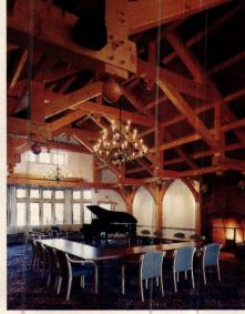
Vermont Timber Works erected this hammer-beam timber-frame building in Stowe, VT.
