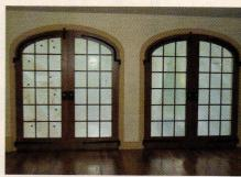
These eliptical arched-top french doors with double pane insulated glass were fabricated by Illingworth Millwork.
