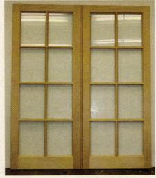
This casement sash window unit was fabricated by Weston Millwork
