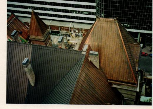
Artificially accelerating the patination of the roof was out of the question. "At Heather & Little, we receive numerous requests to artificially patina various exterior copper components, but in our experience the best protective process is by natural patina – just let it happen the way nature intended it to be," says Forbes.
