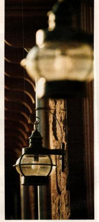
Restored cornice brackets support new copper gutters. Exterior fixtures came from Hanover Lantern of Hanover, PA.
