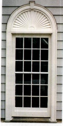
This reproduction 12/12 window with fan was fabricated by Architectural Components.
