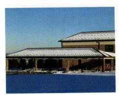
Large, forward-mounted polycarbonate snowguards from Snoblox were used to prevent dangerous movement of snow and ice on this metal roof.
