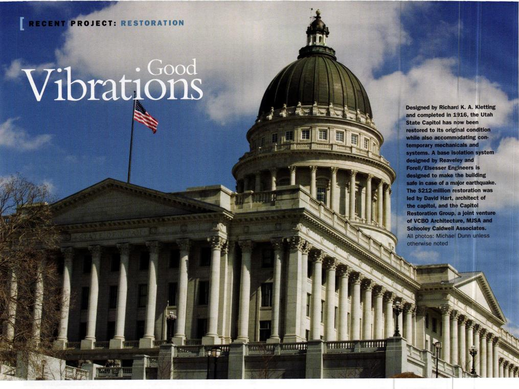
TAKE A 320,000-SQ.FT., 168 million-lb. historic reinforced-concrete capitol with a 226-ft. tall copper-covered dome and shake it around a bit and what happens? Not that much, according to Reaveley Engineers of Salt Lake City, because a comprehensive, one-of-a-kind seismic upgrade has just been installed as part of a multi-year multi-million dollar historic preservation effort.
