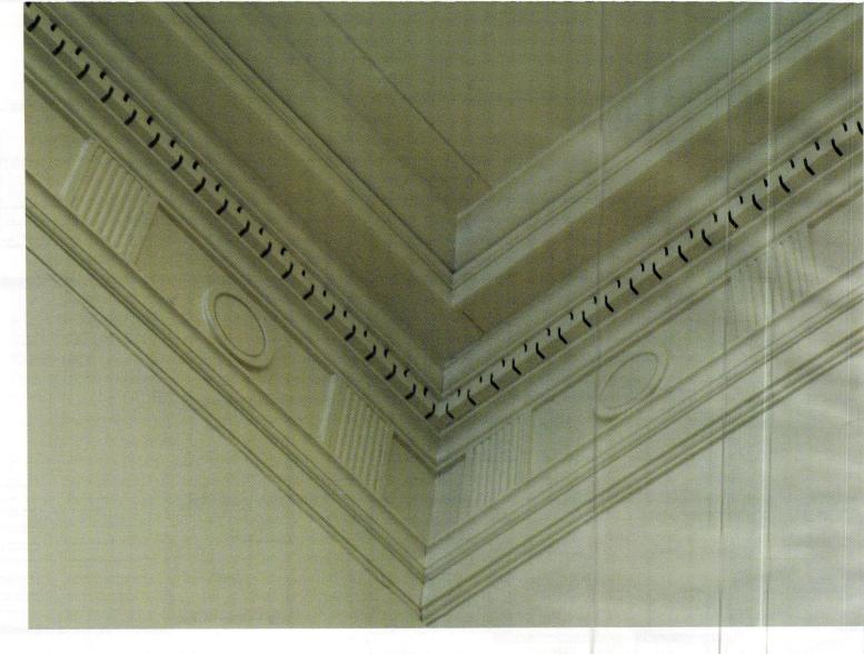
Greek revival cornice work was discovered above a suspended ceiling in the courtroom during construction, and incorporated in the final design.
