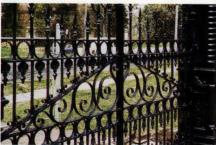
This wrought- and cast-iron entry gate was restored by Architectural Iron Co.
