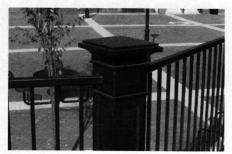
This custom cast-iron stanchion was fabricated by O.K. Foundry.
