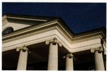
This fiberglass exterior cornice and these GFRC Scamozzi columns were supplied by Architectural Columns & Balustrades by Melton Classics.
