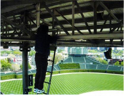
Seven Bird-X UltrasonX units and seven Super BirdXPeller PRO units were installed in the trusses under the upper deck roof overhang and in the lower deck corners of Chicago's Wrigley Field to repel pigeons. Photo: courtesy of Bird-X Inc.
