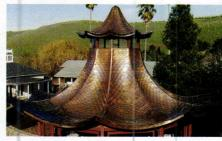
Vulcan Supply custom fabricated the shingles for this copper pagoda in its Vermont shop before completing the installation on site
