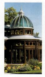
This glass and leadcoated copper dome was designed and constructed by Tanglewood Conservatories for a naturally stained mahogany conservatory.
