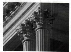
DeAngelis Iron Work supplied and installed 12 cast-iron capitals for the exterior restoration of the Massachusetts State House.
