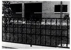
The scroll work in this section of fencing from King Architectural Metals was forged and hot-hammered at the ends
