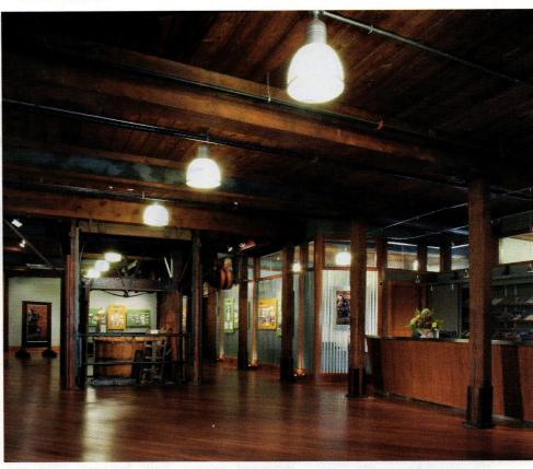
New walls don't touch the columns or ceilings and mechanicals and wood subfloors are exposed, so the interior retains its industrial atmosphere. Photo: Matt Wargo
