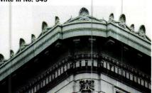
Towne House Restorations replaced the terra-cotta elements on this building with new elements made of cast stone and fiberglass-reinforced concrete.
