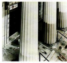
K&E Chemical developed Klenztone, a cleaning formula that penetrates the pores of a masonry surface so that dirt can be released and washed away.
