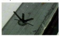
Birdmaster's Trident bracket supports three stainlesssteel cables on a roof parapet.
