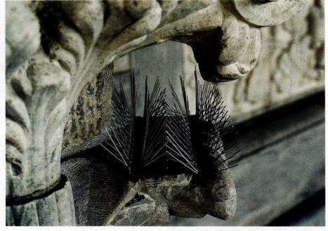
Nixalite of America, Inc., offers eleven different bird-spike models, each providing different capabilities and features. All perform the same service: the effective and humane control of pest birds by rendering a roosting or nesting area uninhabitable. Photo: courtesy of Nixalite of America. Inc.
