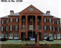
The Durable Slate Co. installed a new double-lock, standing-seam copper roof with vented ridges and hips on the Parish National Bank in Slidell, LA, after it was damaged by Hurricane Katrina.
