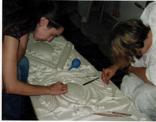
As masters for the GFRC were prepared, plaster models for the rubber molds were meticulously sanded and scraped.
