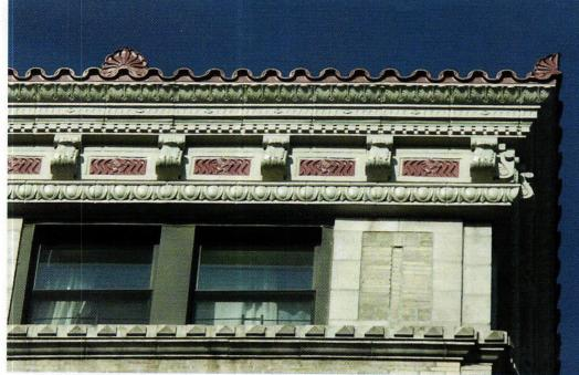
The terra-cotta cornice at 327 Central Park West in New York City is actually a replication in FRP, produced by Architectural Fiberglass Corp. Both colors were molded into the fiberglass, which is lightweight enough to permit the firm to produce numerous "terra cotta" components in single, modular units measuring 6 ft. long and weighing less than 150 lbs. Photo: courtesy of Architectural Fiberglass Corp.
