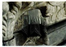
Nixalite bird-control spikes were used on the large, ornate columns under the cornice and pediment of the South Australia Parliament Building in Adelaide, Australia.
