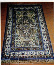
Native Tile & Ceramics creates its "rug" flooring patterns using processes such as Cuerda Seca or Resist Line.
