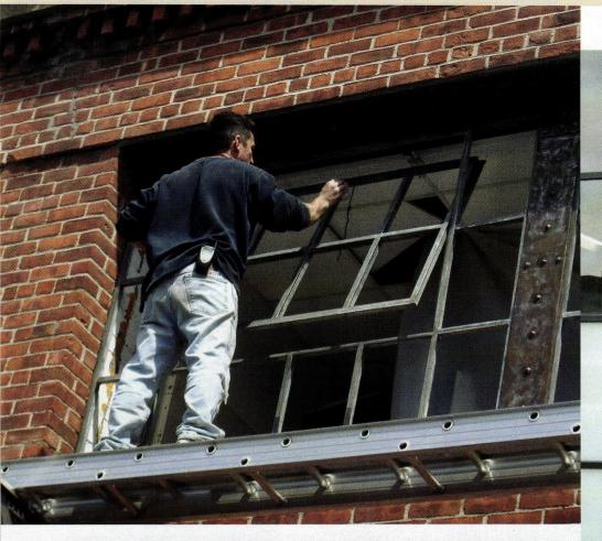
Some of the windows were operational and required only replacement <sup>1</sup>/<sub>4</sub>-in. laminated glass, stripping and painting; others were permanently open.
