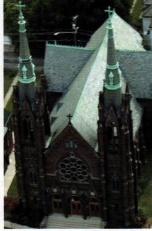
The Durable Slate Co. repaired the slate roof and replaced copper valleys, ridge roll, the copperwork at the base of the steeples and the custom-fabricated copper gutter system for this century-old church and rectory in Ohio.
