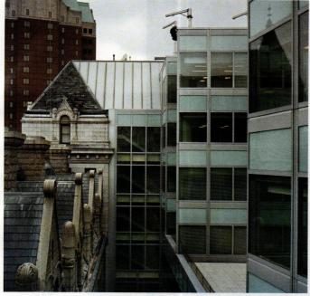
Above: A four-story, U-shaped, painted-aluminum and glass curtain wall encloses the U.S. Attorney's Office, one of the four tenants in the building. Kliment & Halsband designed it to meet the Secretary of the Interior's Standards, clearly contrasting new and old. The height of the addition does not exceed the existing roof line so it can not be seen from the street.
